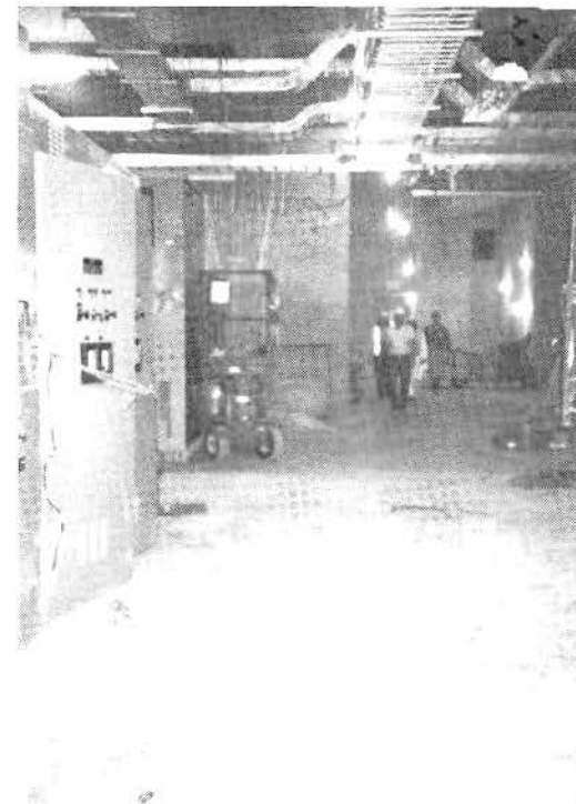
TRANSFORMERS AND CABLE TRAYS BEING INSTALLED IN THE TRACTION POWER SUBSTATION, ROOM #63, HOME SAVINGS BLDG.
