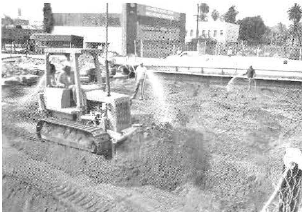
BACKFILL OVER STATION ROOF IN PREPARATION FOR WESTLAKE AVE. DETOUR
