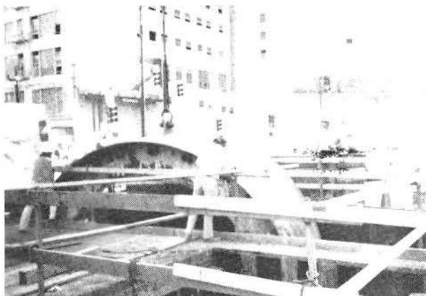
REMOVING FRONT SECTION OF TUNNEL SHIELD AFTER AR SOUTH TUNNEL EXCAVATION
