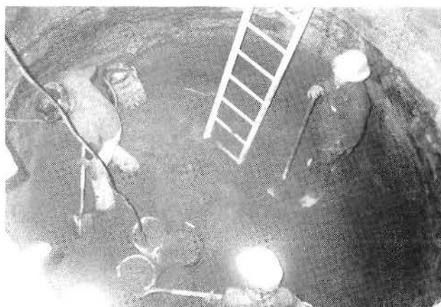
EXCAVATION OF PUMP STATION SUMP
