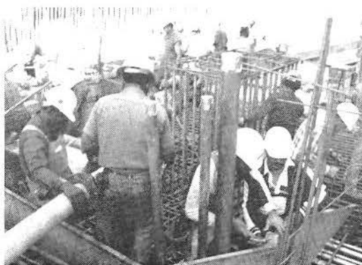
WORKERS GETTING FORM, REBAR AND UTILITIES READY FOR CONCRETE POUR IN LIFT #3A
