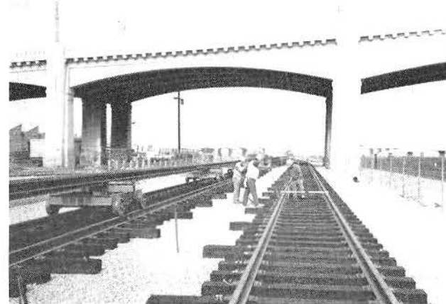
GAUGING AND SPIKING TAIL TRACK TL-1 UNDER SIXTH STREET BRIDGE.
