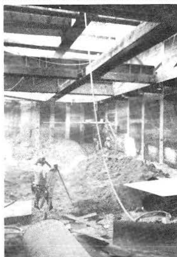
ESTABLISHING THE SOUTHEAST ENTRANCE'S INVERT ELEVATION
