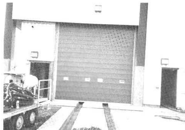
NORTH END OF THE BLOWDOWN AREA AND ENTRANCE TO CONTROL TOWER
