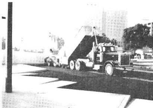
PAVING OF THE LOWER PARKING LOT ON THE WEST SIDE OF THE BAGGAGE HANDLING FACILITY
