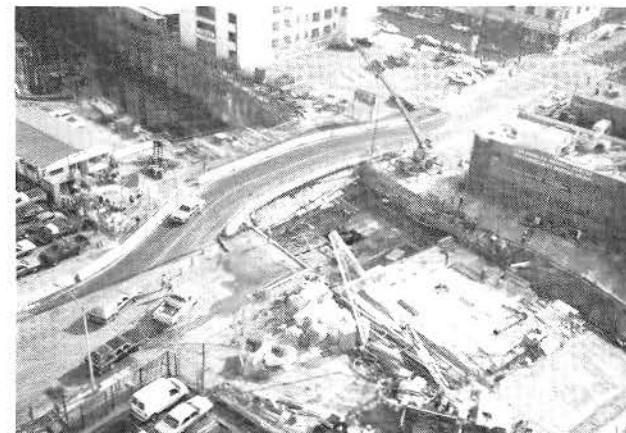
OVERVIEW OF WESTLAKE AVE. DETOUR, OVER STATION STRUCTURE
