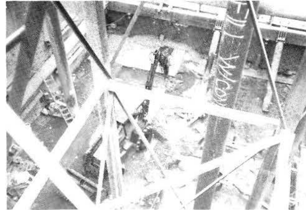
DEMOLITION AND REMOVAL OF CONCRETE PADS AT THE BASE OF ACCESS SHAFT
