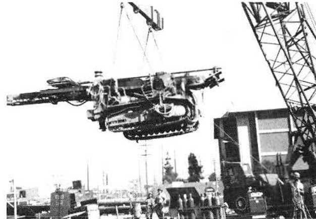
NICHOLSON CONSTRUCTION CO. DRILL RIG BEING LOWERED INTO BOX STRUCTURE FOR TIEBACK INSTALLATION
