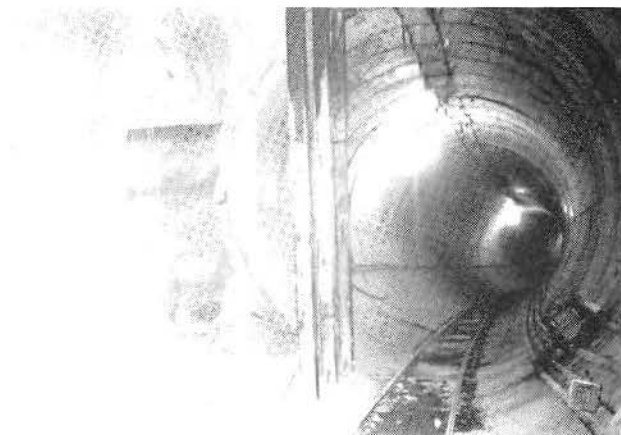
INTERSECTION OF CROSS PASSAGE #7 AND AR TUNNEL
