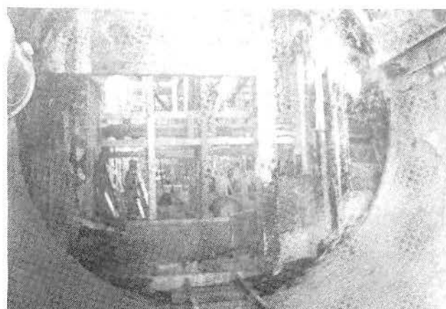
BREAK THROUGH OF AL TAIL TUNNEL INTO A145 STATION
