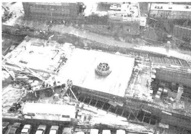
OVERVIEW OF STATION AREA AFTER PLACEMENT OF ROOF CONCRETE, WEST OF WESTLAKE AVE.
