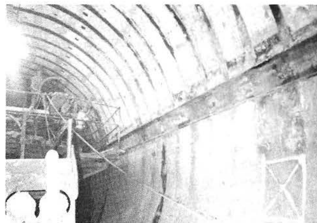
PREPARING AIR TAIL TUNNEL FOR HDPE INSTALLATION
