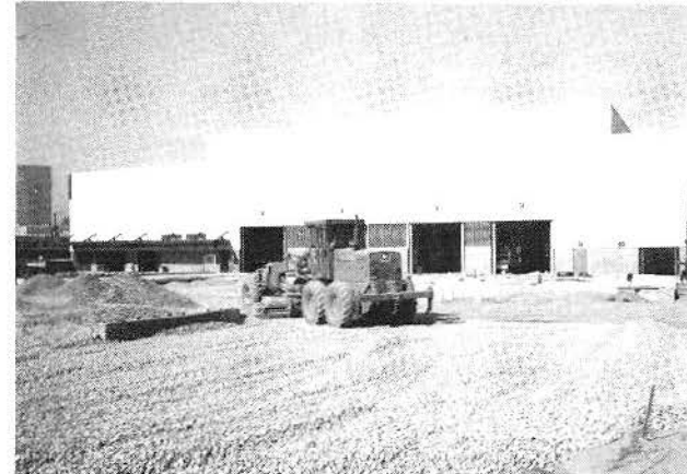
SPREADING BALLAST SOUTH OF MAIN SHOP BUILDING
