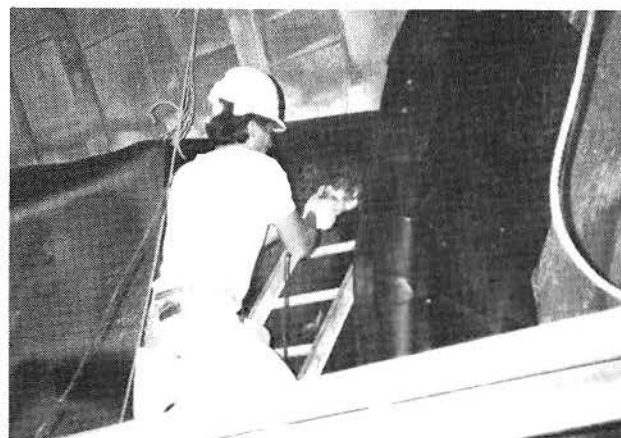
WORKMAN INSTALLING HDPE IN CROSS PASSAGE #9
