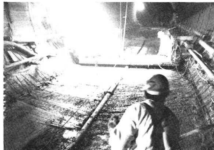
FINISHING OF AL TUNNEL CONCRETE INVERT POUR AT SOUTH END OF TUNNEL
