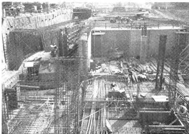
INSTALLATION OF EMBEDDED ITEMS PRIOR TO PLACEMENT OF MEZZANINE CONCRETE AT THE STATION'S WEST END (LOOKING EAST)
