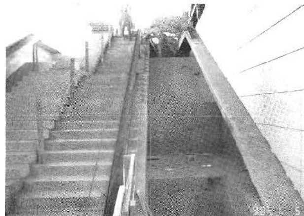
HOME SAVINGS ENTRANCE TO THE METRO RAIL STATION
