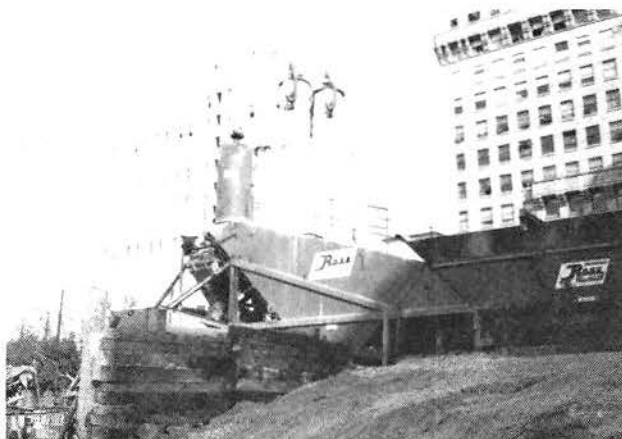
CONCRETE BATCH PLANT AT SITE
