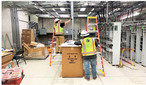
Wilshire/Western Station Systems Installation
