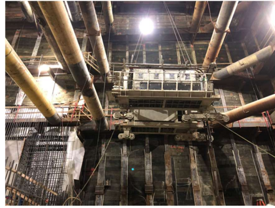
BR TBM Gantry #2 Hoisted to Street Level
