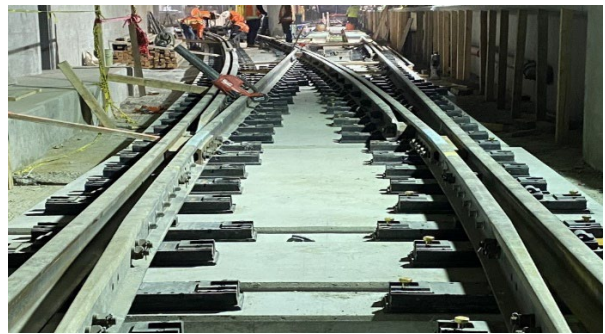
Wilshire/La Cienega Crossover Construction
