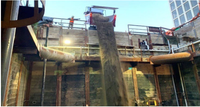
Backfill Activities at Wilshire/Western Interface Chamber
