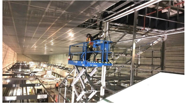
Installing Glazing Frame at Wilshire/La Brea Station
