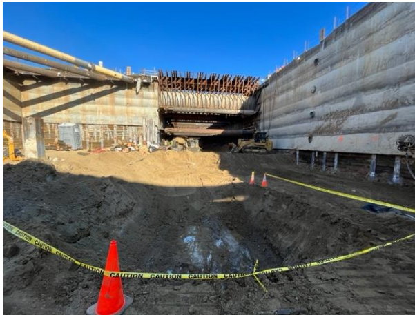
Westwood/VA Station Main Entrance Preparation for Tunnel Dismantling in Excavated Box
