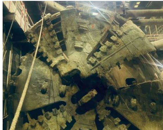
BR TBM Cutterhead Extraction
