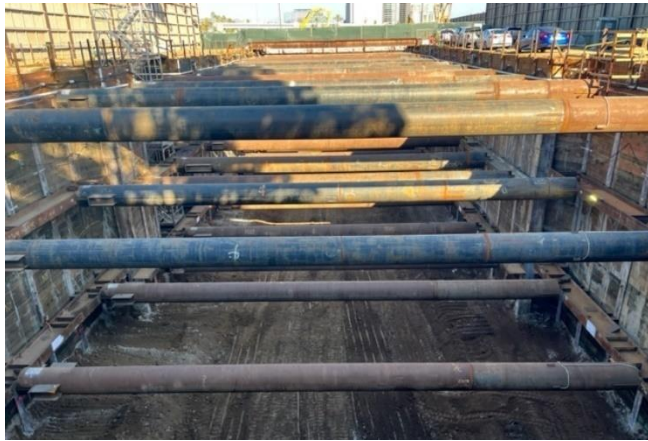
Westwood/VA Station: Level 4 Excavation & Lagging
