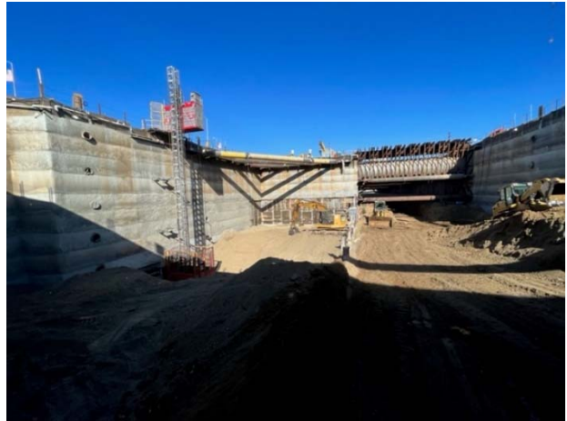
Westwood/VA Station: Lift Installation and Excavation at Main Entrance
