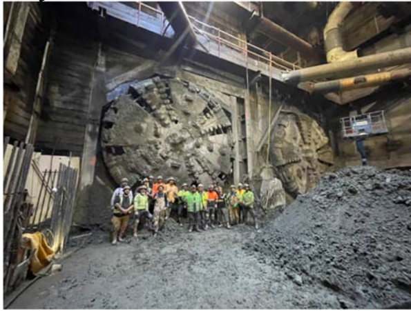
TBM Hole Through at Century City/Constellation Station
