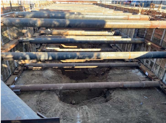
Westwood/VA Station: Struts at Level 3
