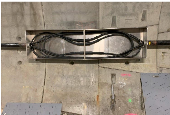
Reach 2 Tunnel (La Brea to Fairfax) Trainway Feeder Installation
