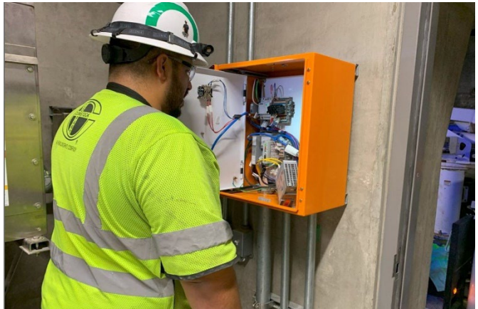
Reach 1 Tunnel (Western to La Brea) Commissioning
