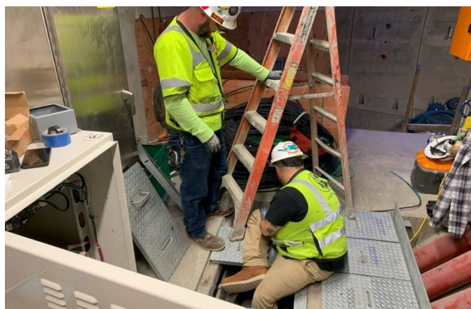
Reach 4 Tunnel Cross Passage Fire Alarm & Intrusion Cabling
