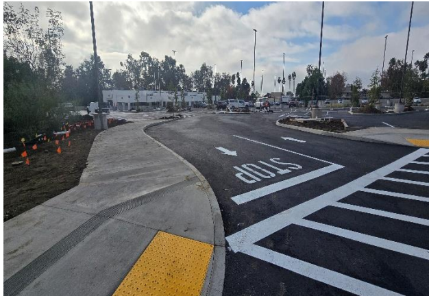
VA Parking: Lot 527 Completed Paving and Striping
