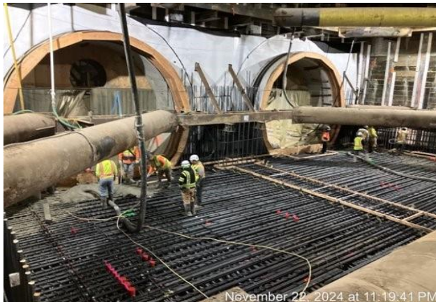
Westwood/VA Hospital Station: Invert Concrete Pour 1 (East End)
