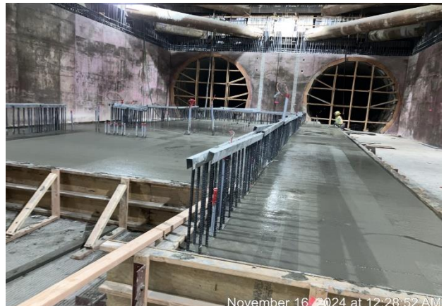
Westwood/UCLA Station: Placing Concrete for Secondary Invert (East End)
