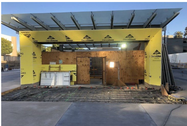
Wilshire/La Cienega Station (Plaza) Main Entrance Structure
