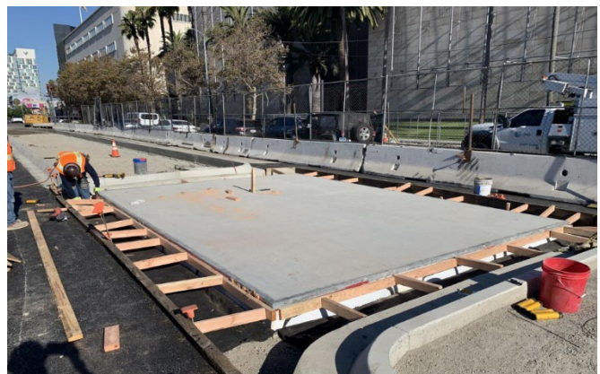
Wilshire/Fairfax Station Permanent Hatch Installation
