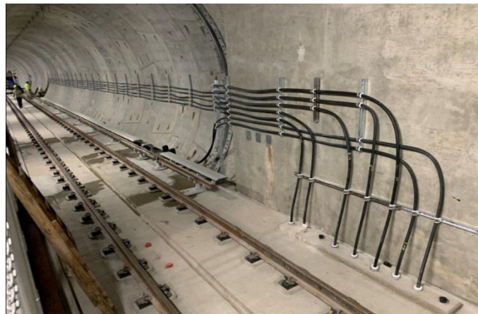
Reach 1 Tunnel (Western to La Brea) Cable Installation
