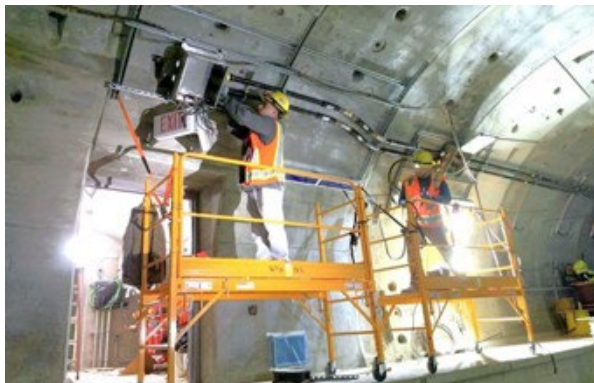
Phenolic Conduit Installation (Reach 2)
