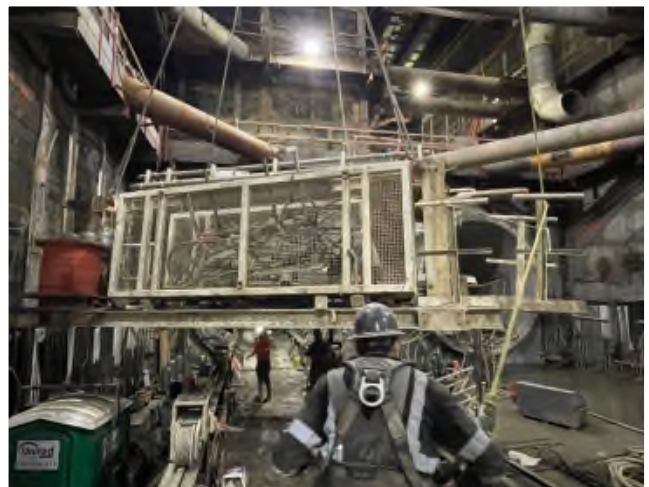
BL TBM Gantry Extraction from Century City/Constellation
