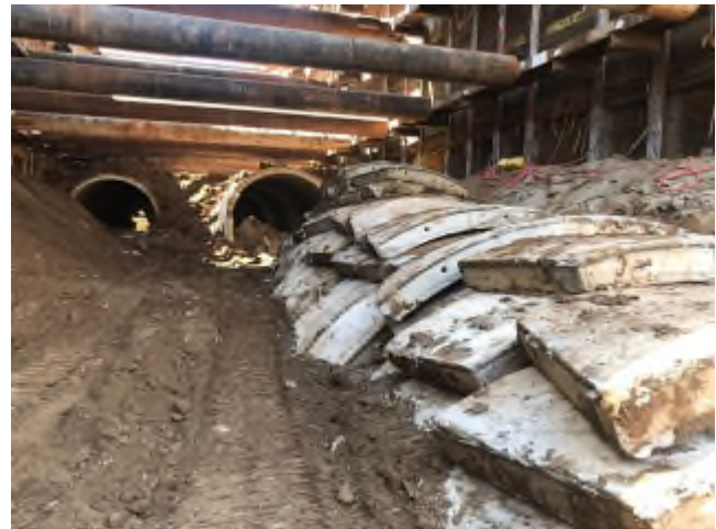
Westwood/VA Hospital Station: Excavation and Tunnel Segment Removal
