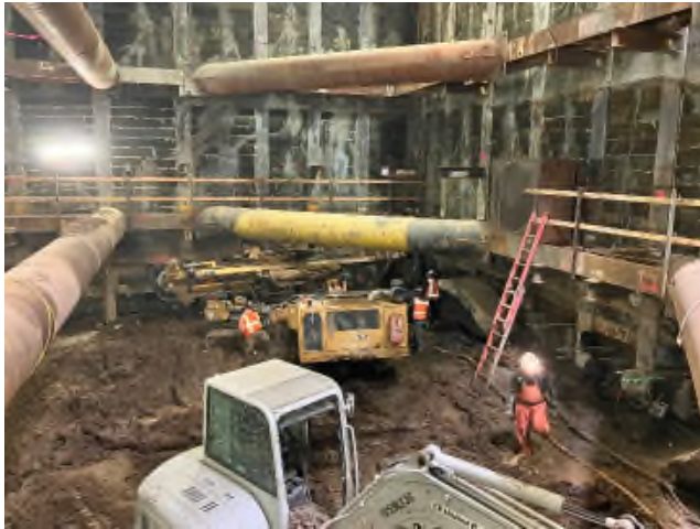
Westwood/UCLA Station: Soil Nail Operation at the West End Wall
