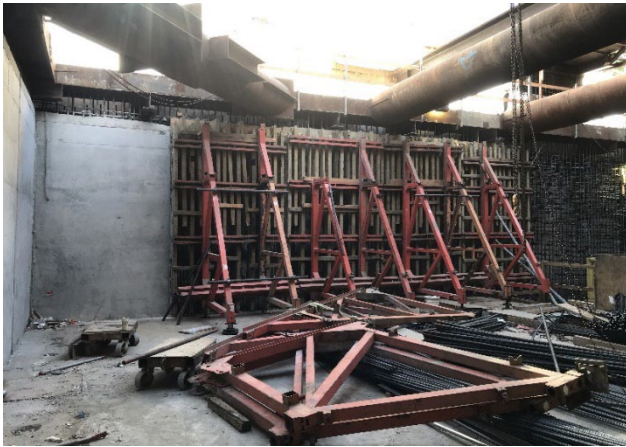
WRS Station Entrance Exterior Wall Forms
