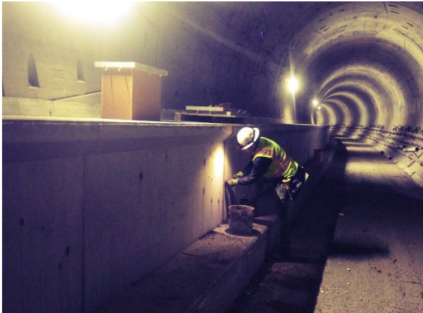
Tunnel Walkway Patching in BL Reach 5
