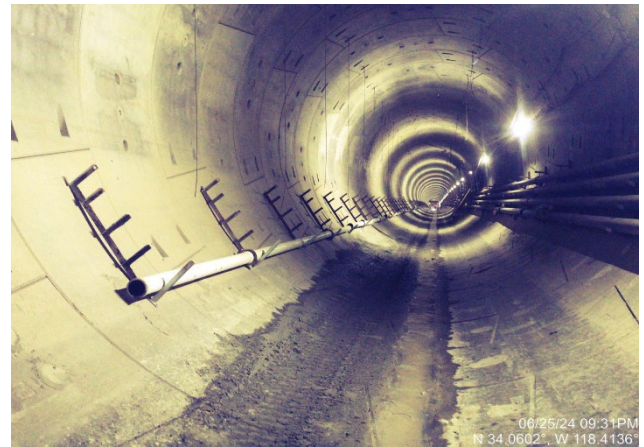
Tunnel Removal of Utility Lines
