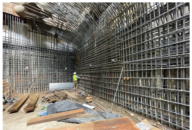
CCCS Rebar at East Side Exterior Wall Concourse Level
