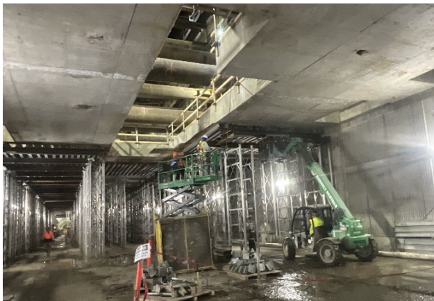
CCCS Falsework Stripping Concourse Level
