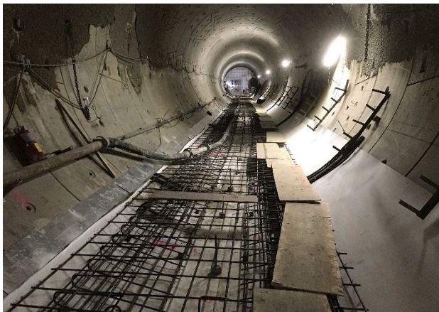
Tunnel Invert Rebar Installation
