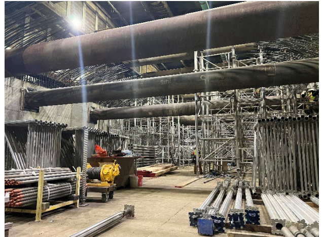
WRS West Highbay Walls-Falsework for Roof Deck
