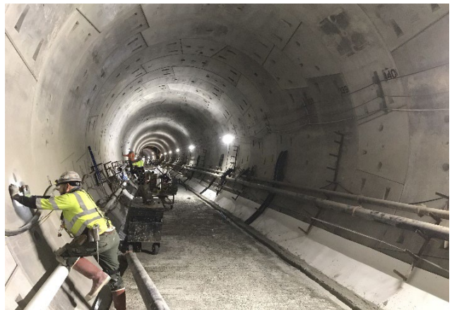
Relocating Utilities to Make Way for Walkway
