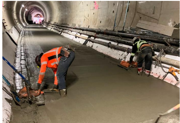
Tunnels: First Stage Invert Concrete Pour (Reach 7)
