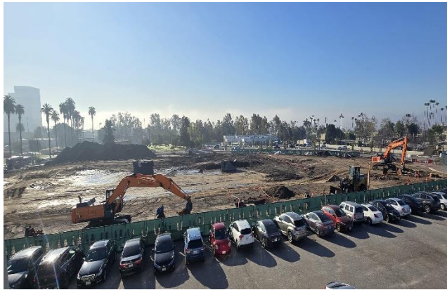
VA Parking Structure: Completed Preparations of Building Base Pad Material for New Structure
