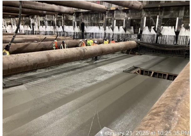
Westwood/UCLA Station: Concourse Slab Placement (Section 2)
