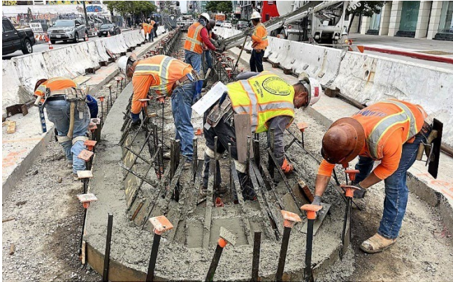
Wilshire/Western Station Median Restoration
