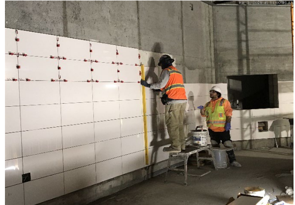
CCS Room No. 61 Tile Installation
