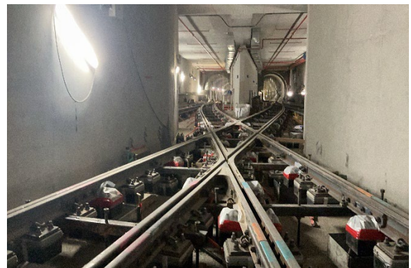
CCS DXO Track Installation
