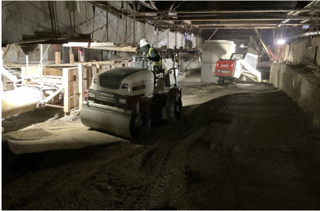
CCS Ongoing Roof Backfill and Compaction
