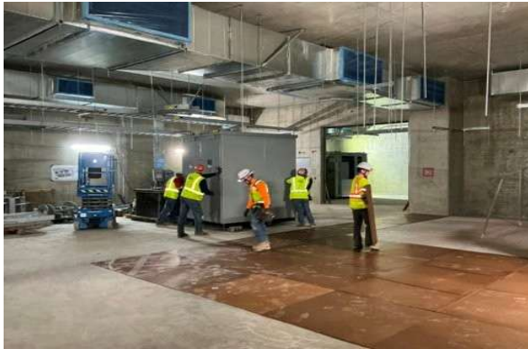
Westwood/VA Hospital Station: Dielectric Flooring Installation in Southern California Edison Metering Switchgear Room
