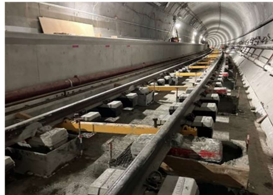
Track/Tunnels: LVT Block and Running Rail Installation in Reach 6
