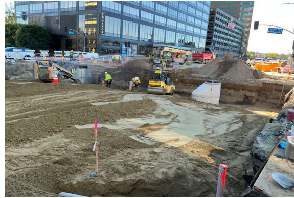
Westwood/UCLA Station: Deck Removal and Backfill on Wilshire Blvd
