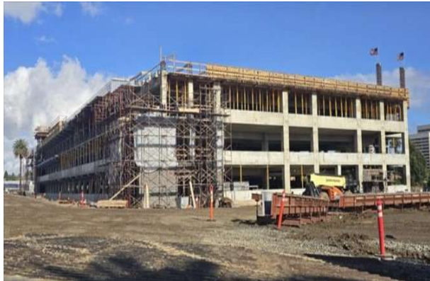
VA Parking Structure: Level 4 and 5 Deck Construction
