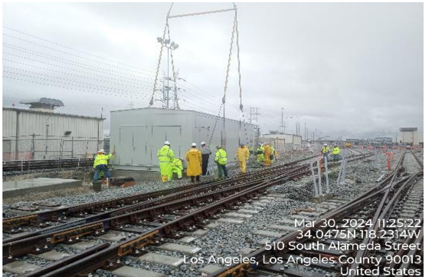
South Yard – Ladder Track installing bonded joint bars
