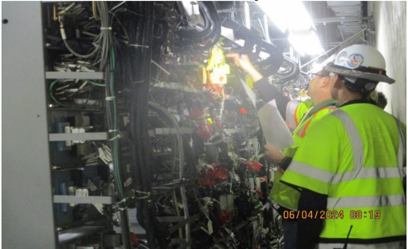
Test , cut, lug, & land 500 Kcmil contact rail jumpers on 3 rd rail
