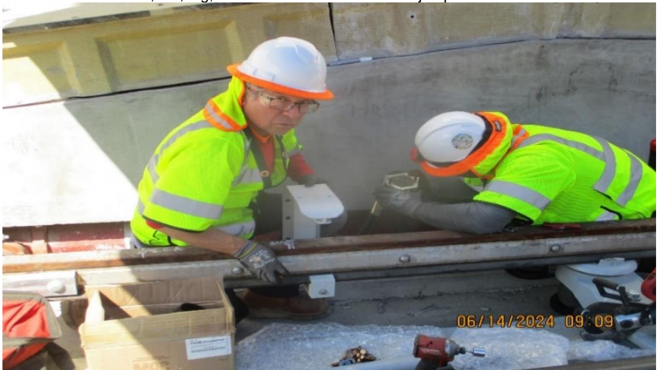
Test , cut, lug, & land 500 Kcmil contact rail jumpers on 3 rd rail
