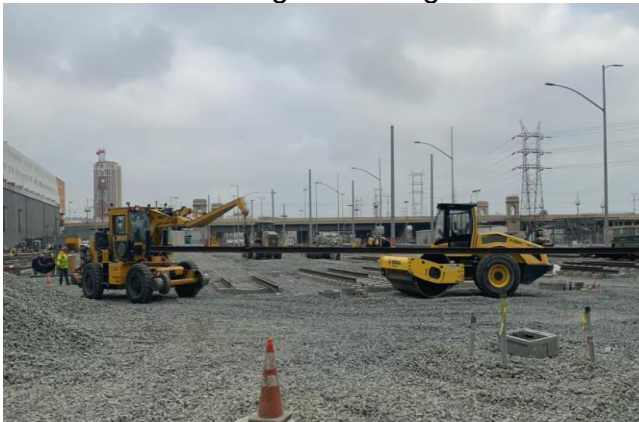
Pulling Rail strings
