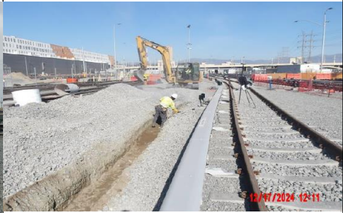
Communication ductbank excavation
