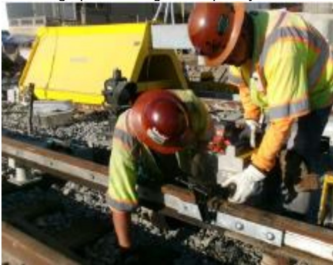
Setting up for drilling CR's splice joint bars
