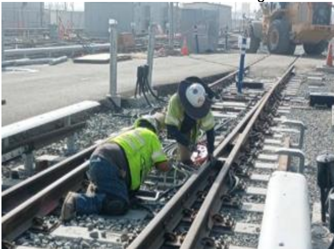
Cad Welded Track Bonding
