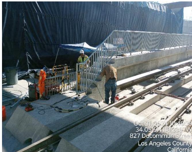
Repairing cable troughs in the Portal
