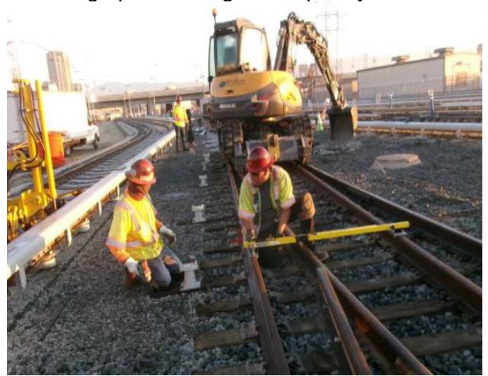
Setting up for drilling CR's splice joint bars
