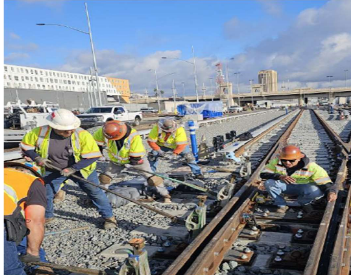
Manually lifting entire Switch with Track Jacks
