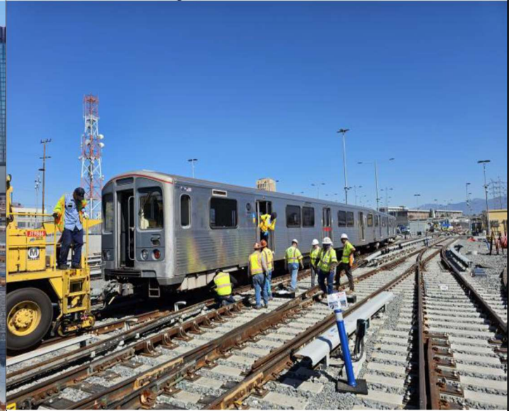
Throwing Switches for the test train
