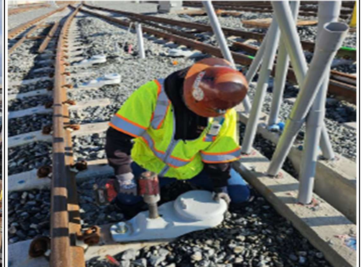
Installing Pedestal Mounts For 3rd Rail
