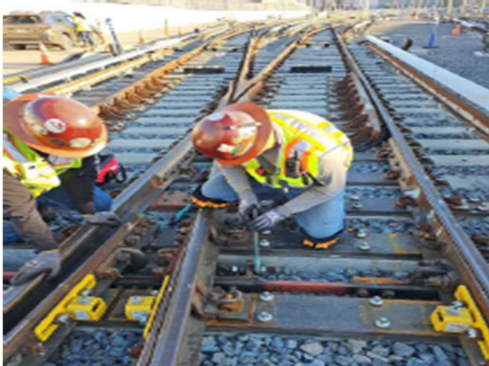
Manually lifting entire Switch with Track Jacks
