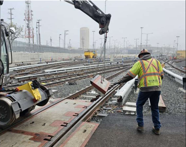
Crossing Panel installation
