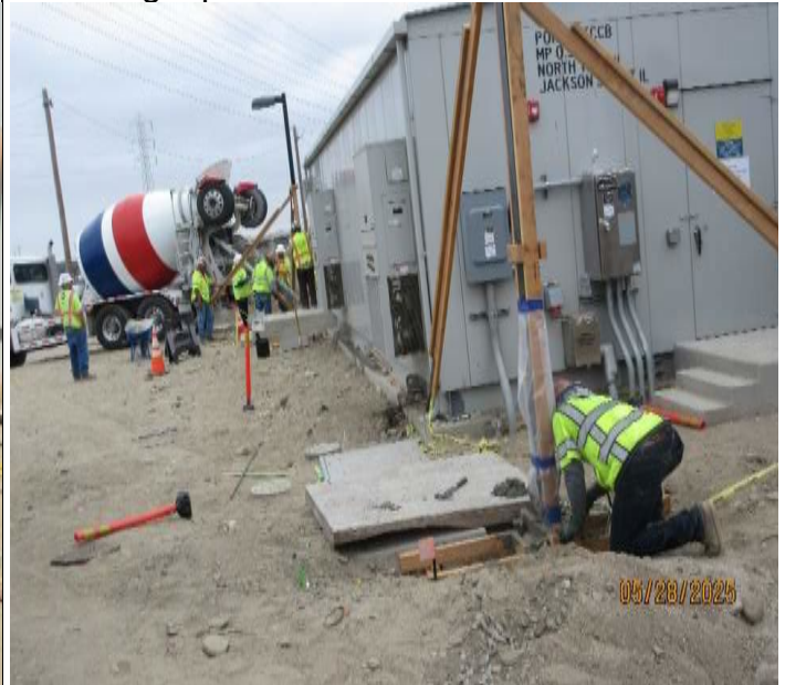
AL 10/10a underdrains with cleanout risers
