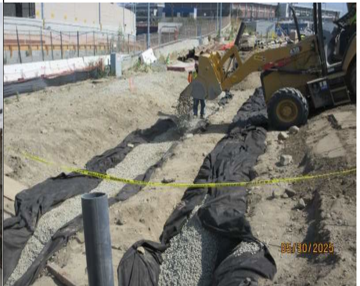
AL 10/10a underdrains with cleanout risers
