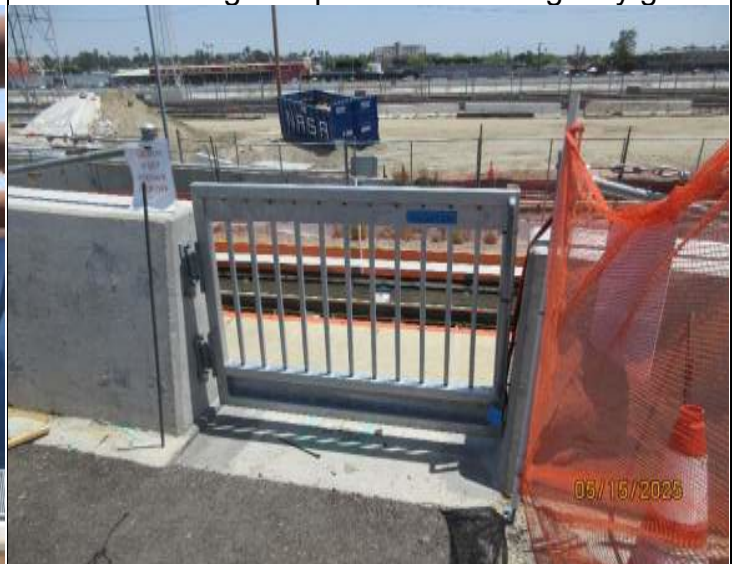
West retaining wall pedestrian emergency gate
