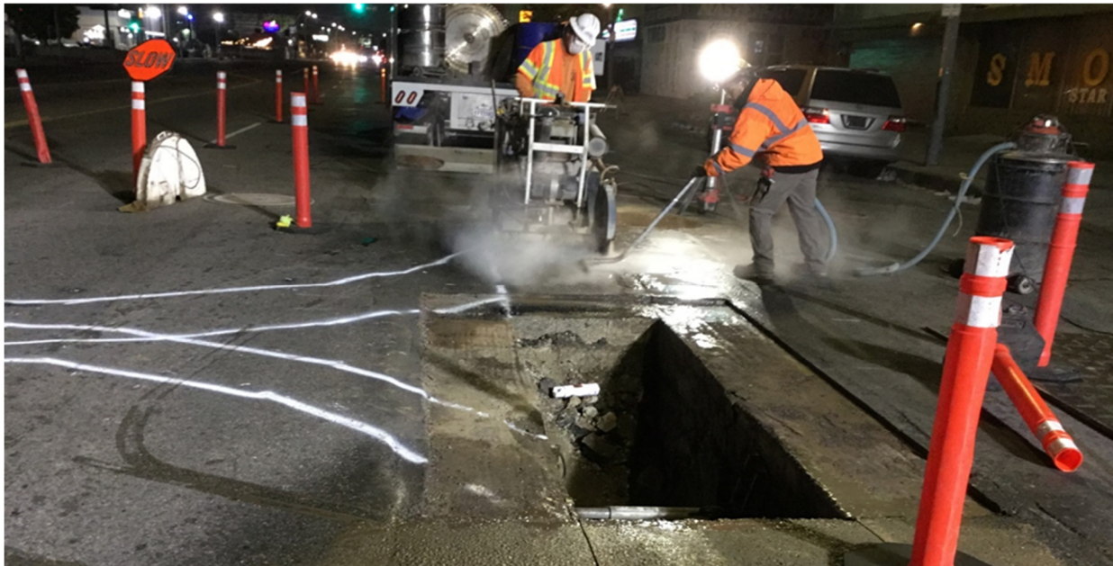
WA Rasic has Tom Grbvac and Sons saw cutting asphalt
