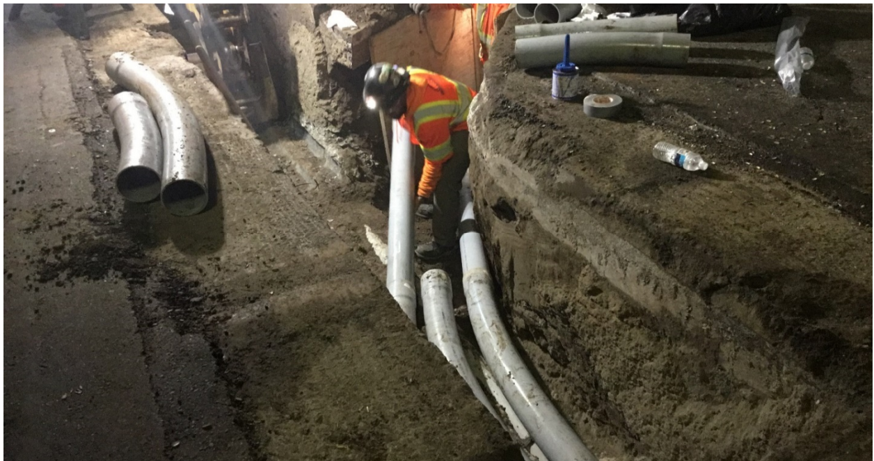
WA Rasic re-routing (3) 5" conduits and excavating to expose existing conduits
