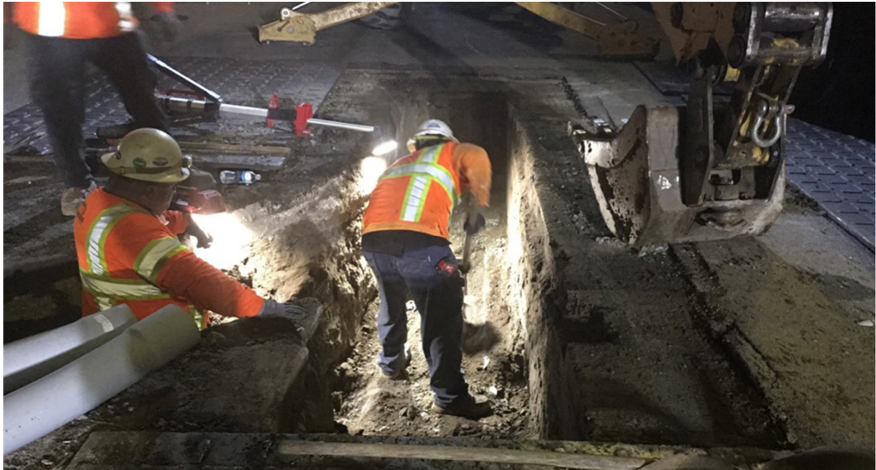
WA Rasic excavating with pneumatic jackhammer to expose existing conduit
