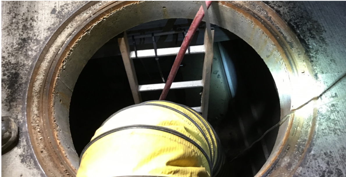
WA Rasic providing mandrel between vaults 6924 and 6940
