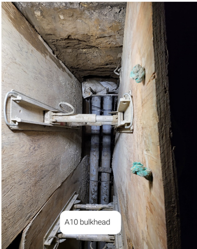
WA Rasic: Lateral A10 bulkhead installed, ready for encasement
