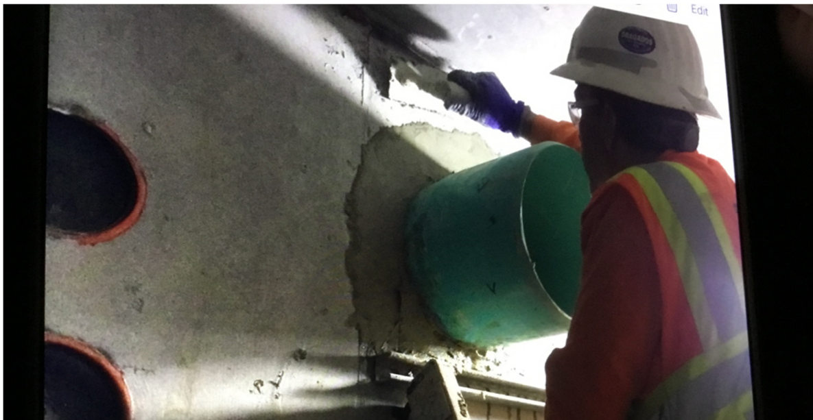
WA Rasic working inside vaults 6900 and 6924. Sealed end of conduits.
