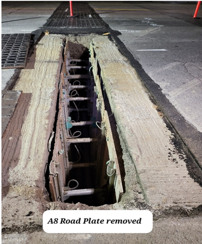
WA Rasic: Road plate removal and setting up for work
