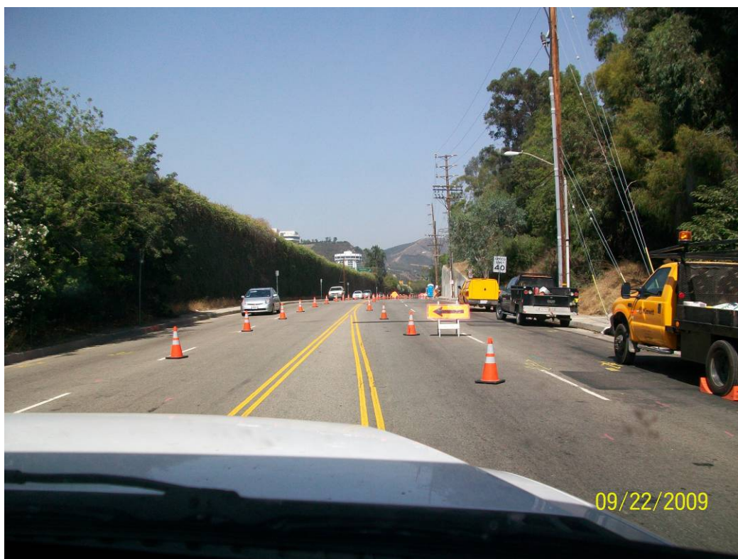
Maintenance of traffic (MOT) Sepulveda Blvd.
