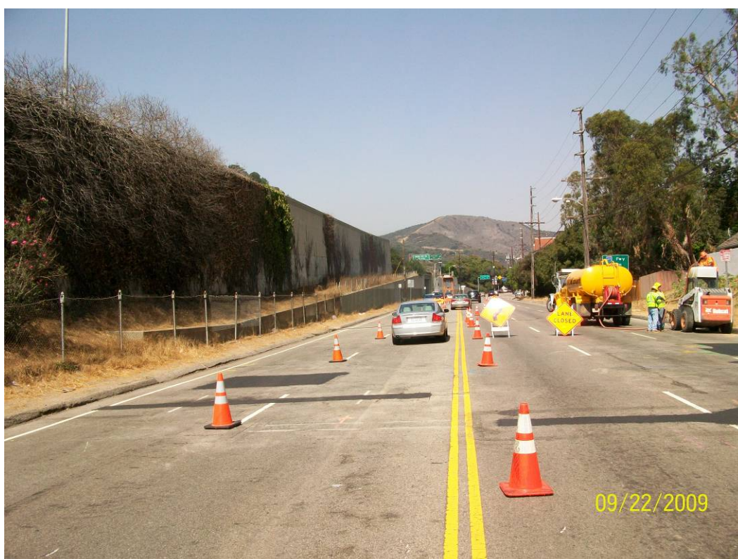
Maintenance of traffic (MOT) Sepulveda Blvd.
