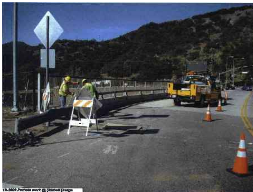
Pothole work at Skirball Bridge.
