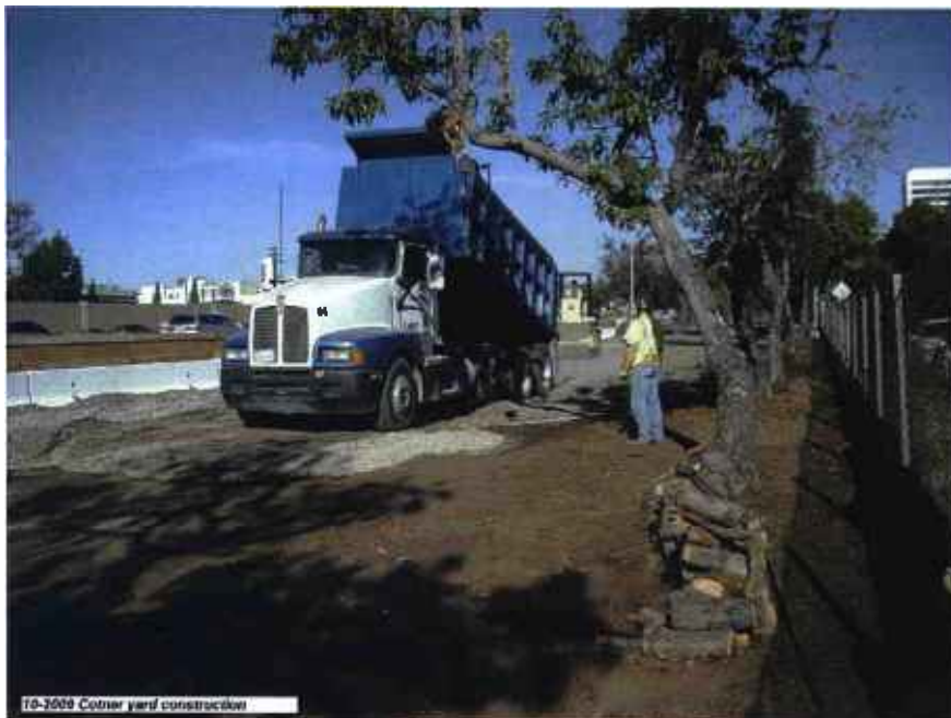
Cotner Yard construction.
