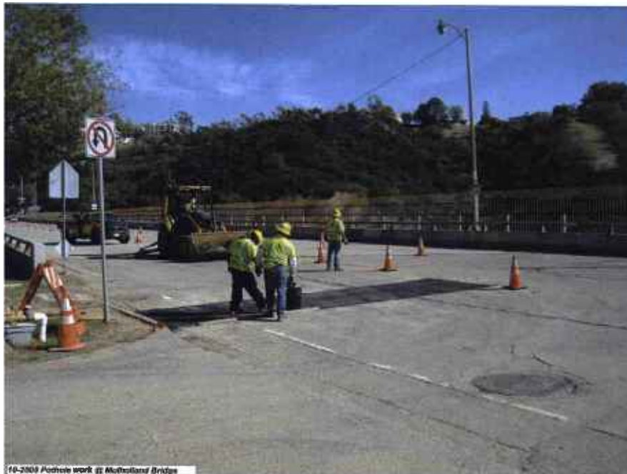
Pothole work at Mulholland Bridge.
