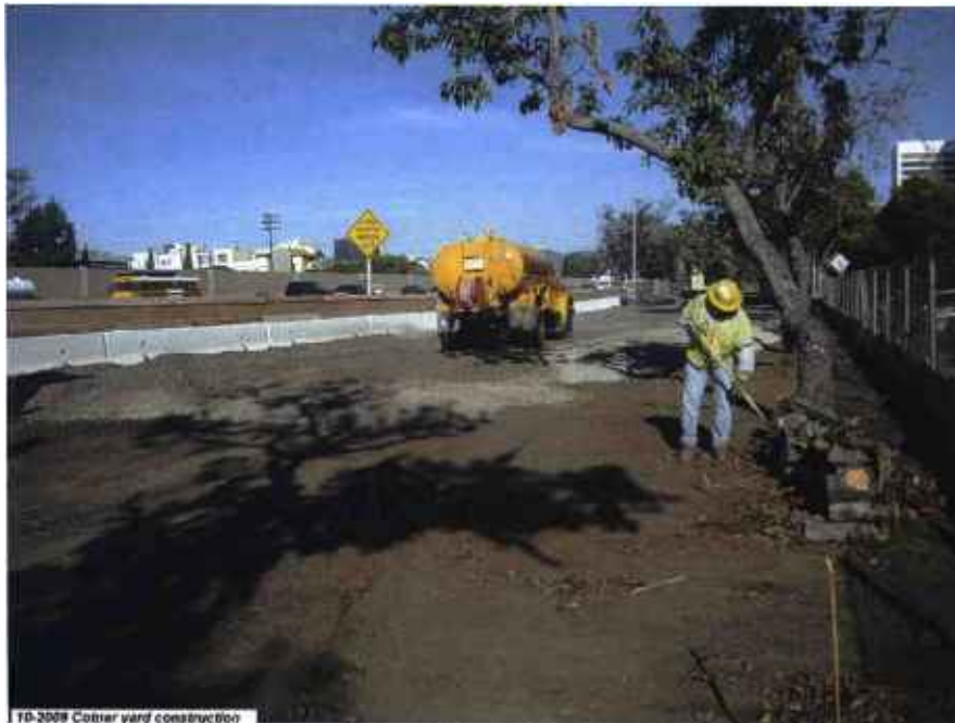
Cotner Yard construction.
