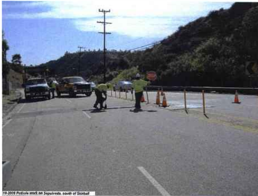
Pothole work on Sepulveda south of Skirball.
