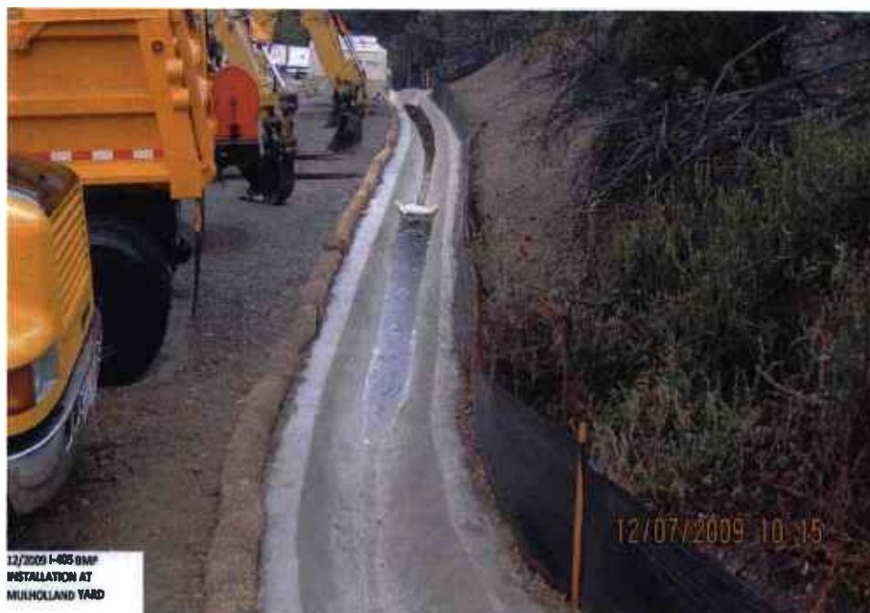
I-405 BMP installation at Mulholland Yard.
