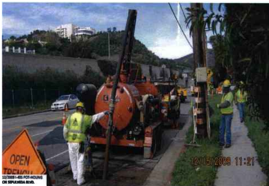
I-405 pot-hole set-up on Sepulveda Blvd.
