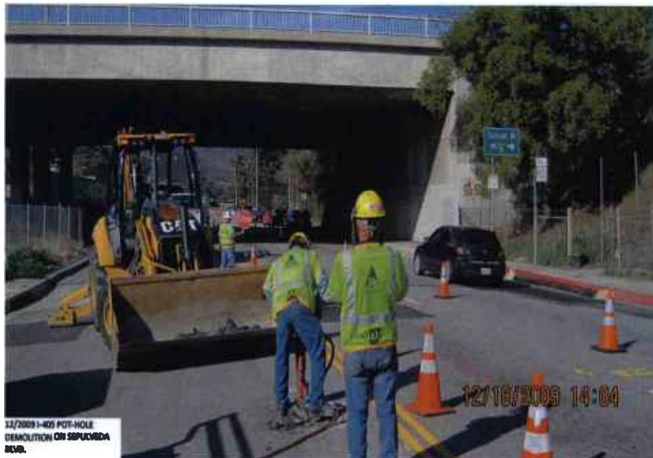
I-405 pot-hole demolition on Sepulveda Blvd.
