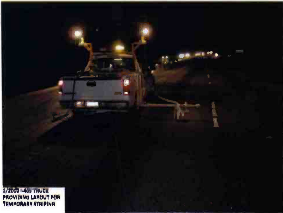
Truck providing layout for temporary striping.
