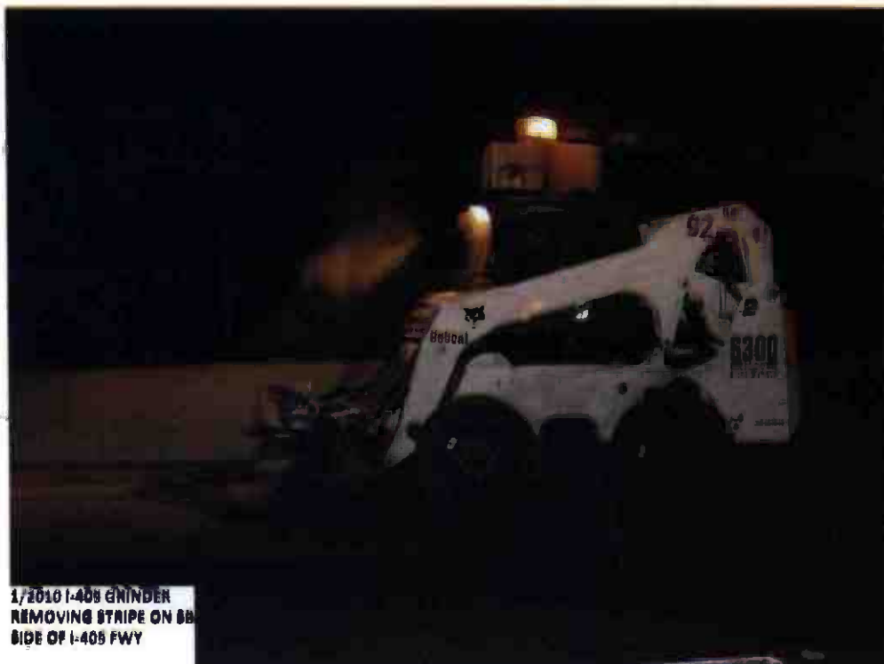
Grinder removing stripe on SB side of I-405 Freeway.
