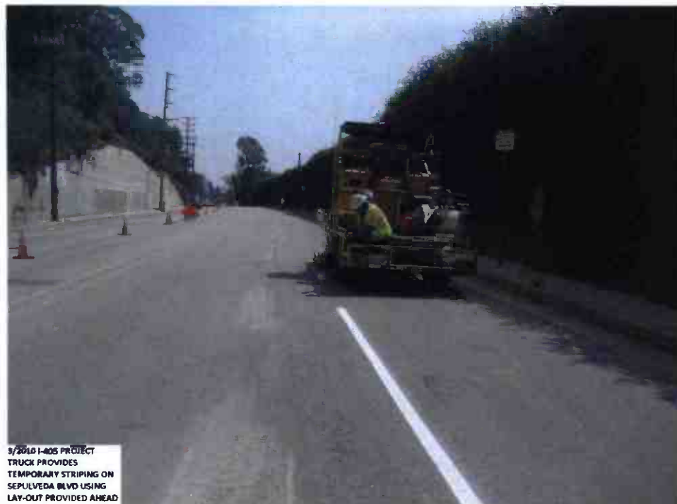
Truck provides temporary striping on Sepulveda Blvd. using lay-out provided ahead.
