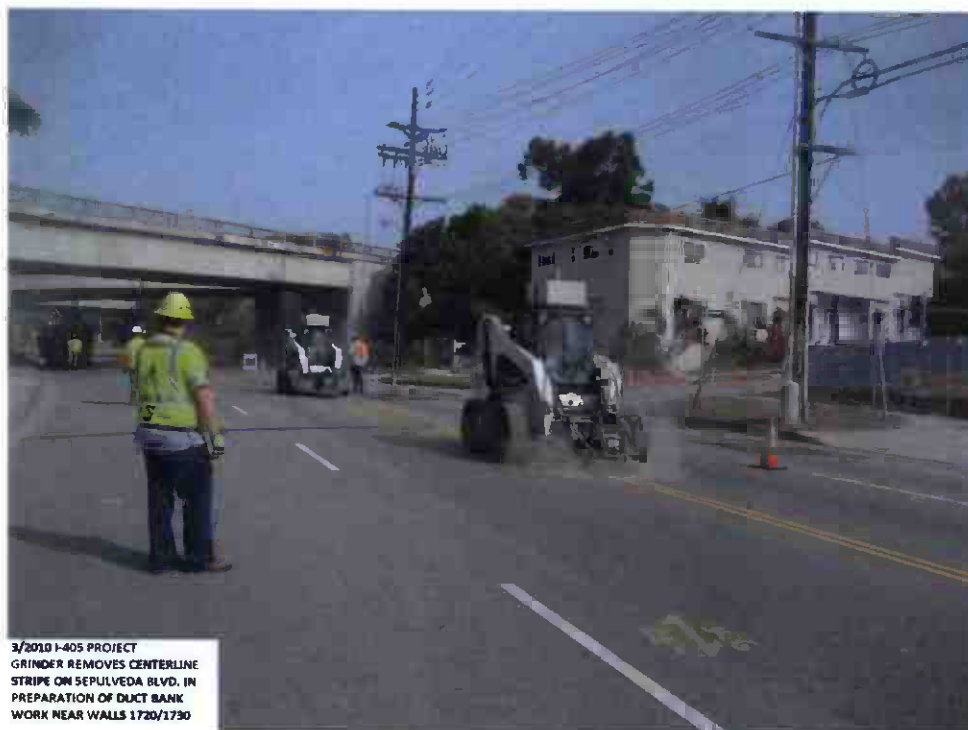
Grinder removes centerline stripe on Sepulveda Blvd. in preparation of duct bank work near walls 1720/1730.
