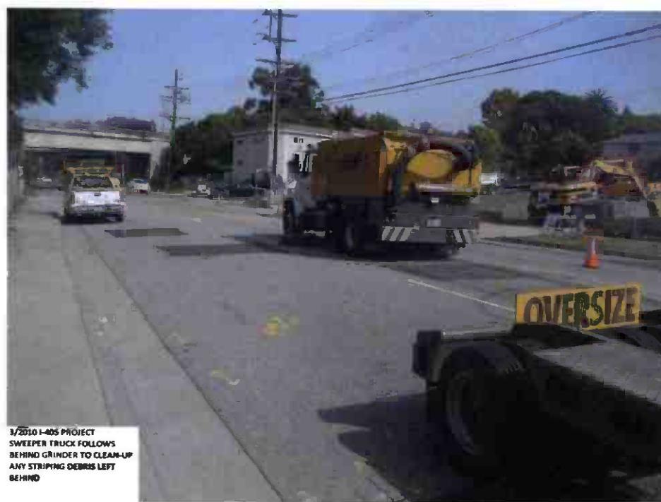
Sweeper truck follows behind grinder to clean-up any striping debris left behind.
