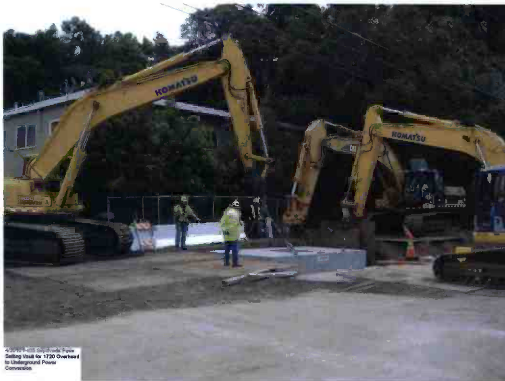
Setting vault for 1720 overhead to underground power conversion.
