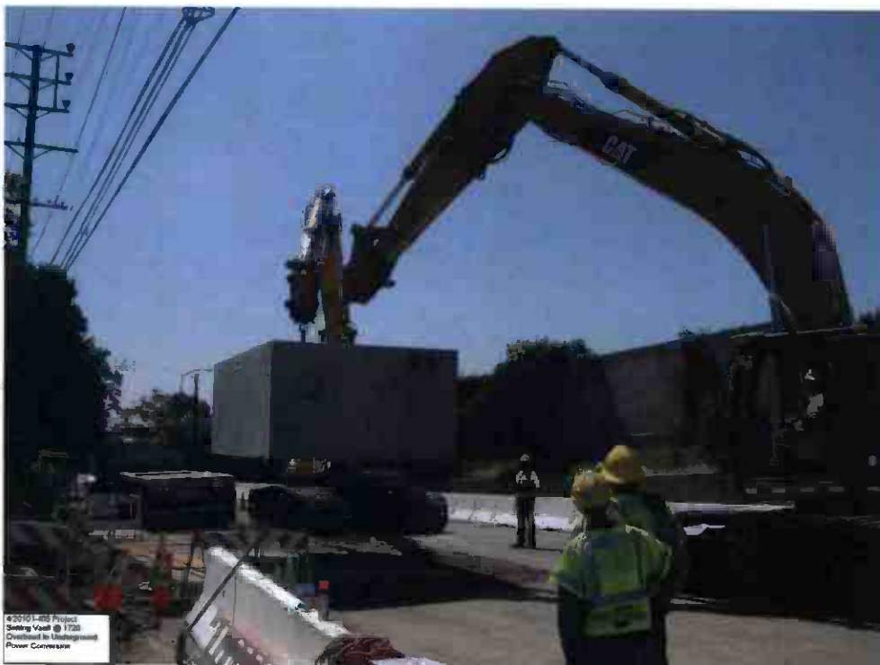
Setting vault @ 1720 overhead to underground power conversion.
