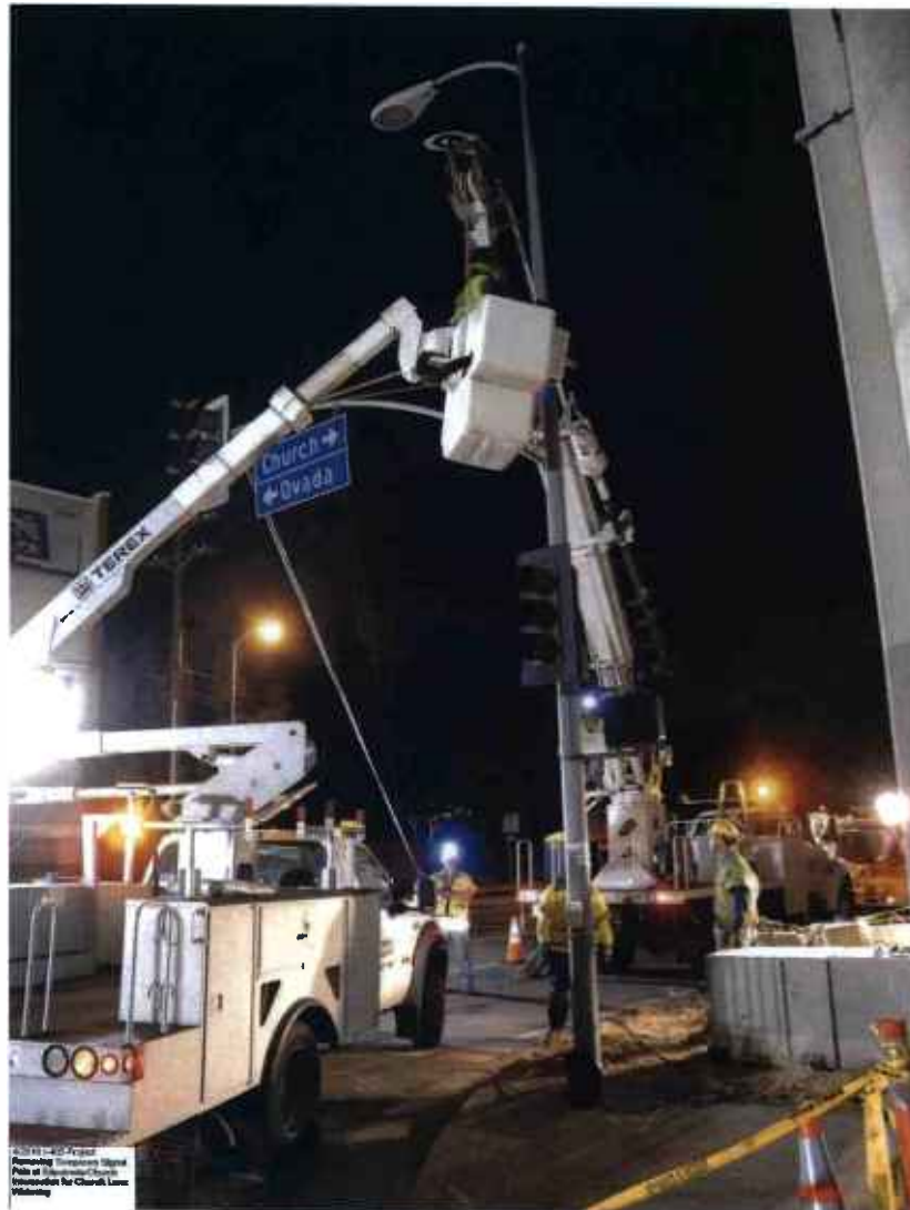
Removing temporary signal pole at Sepulveda/Church intersection for Church Lane widening.
