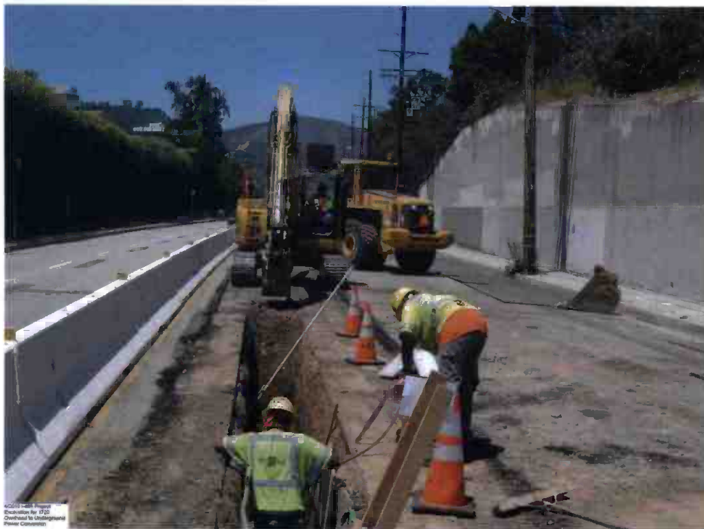
Excavation for 1720 overhead to underground power conversion.
