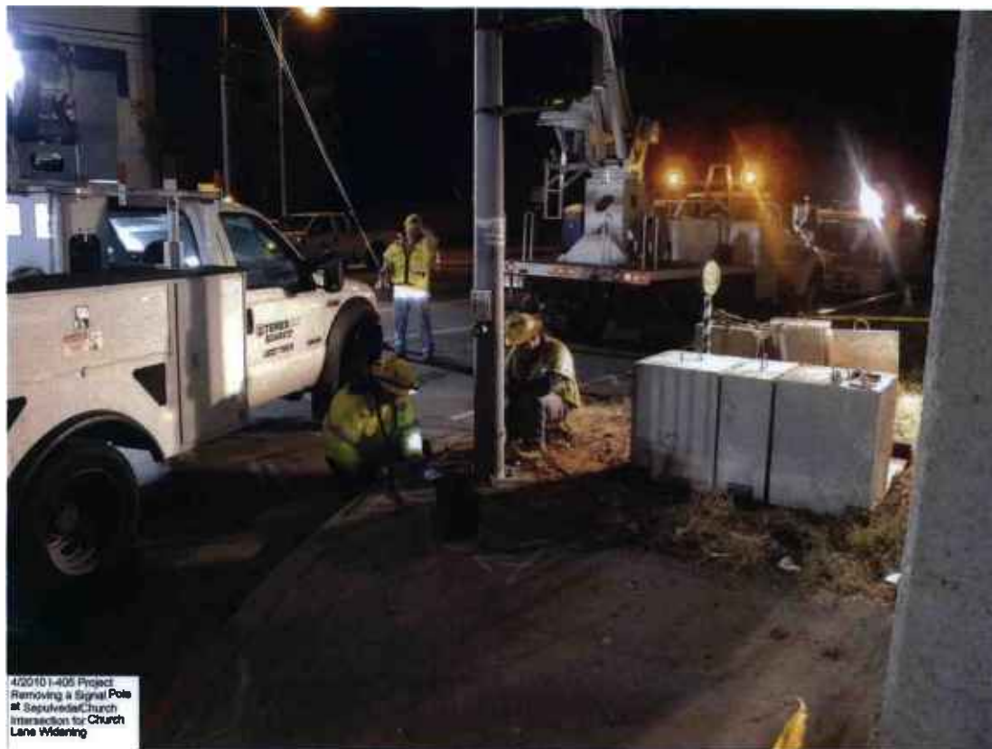
Removing a signal pole at Sepulveda/Church intersection for Church Lane widening.
