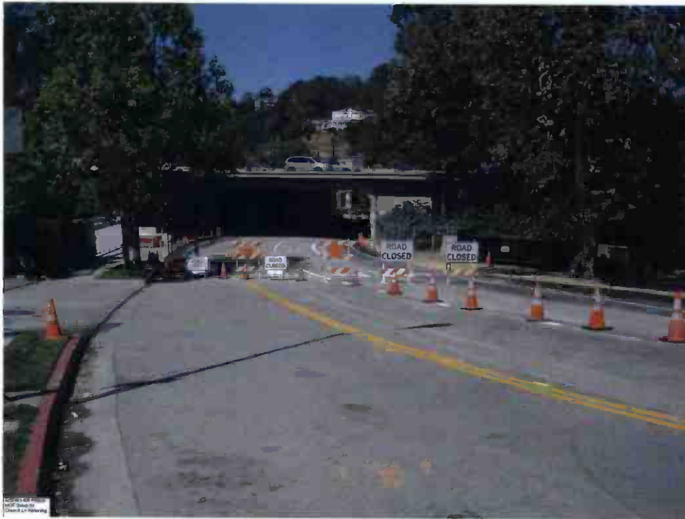
Project MOT setup for Church Lane widening.
