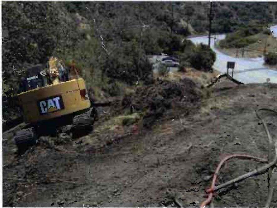
Clear and grub at Wall 1836.
