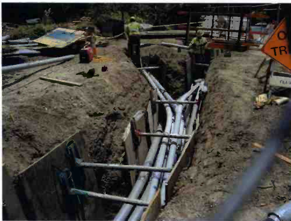
Ductbank on Sepulveda Blvd. at Homedale.
