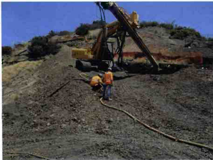
Soil Nail Test at Wall 1836.
