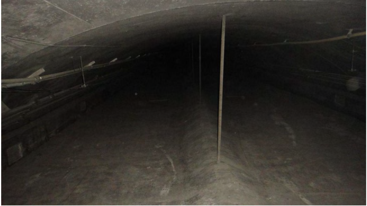
Figure L-6. Visual image of the top of the Chesapeake Bay Tunnel.
