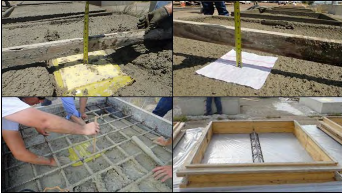
Figure M-3. Construction of slabs with simulated defects.
