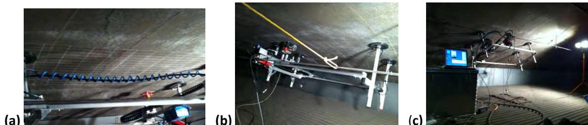
Figure Q-34. HL2: (a) crack running across the test area, (b) NDT scanner mounted on the tunnel ceiling, and (c) scanning of the test area.
