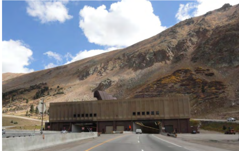
Figure M-16. Eisenhower Memorial Tunnel, Colorado.
