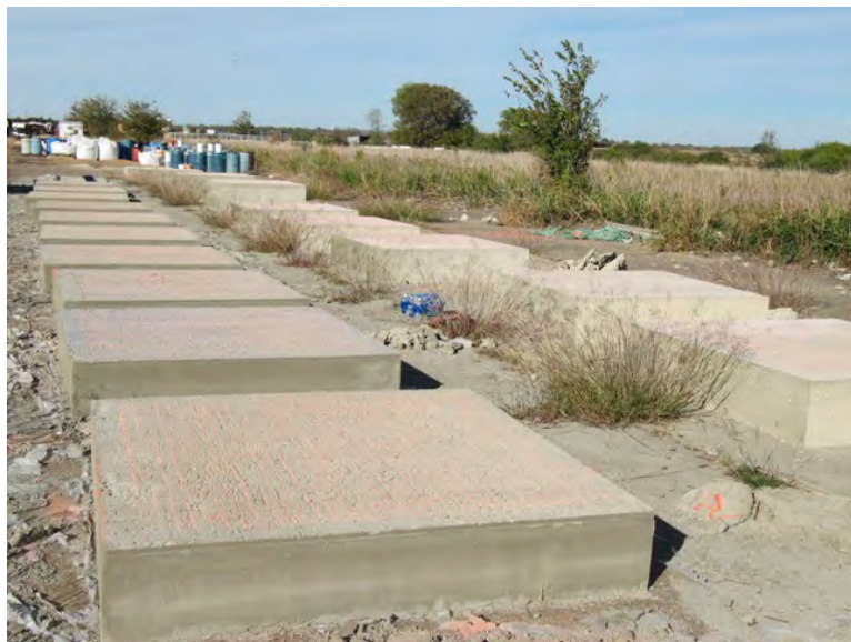
Figure U-2. Overall view of TTI slabs.
