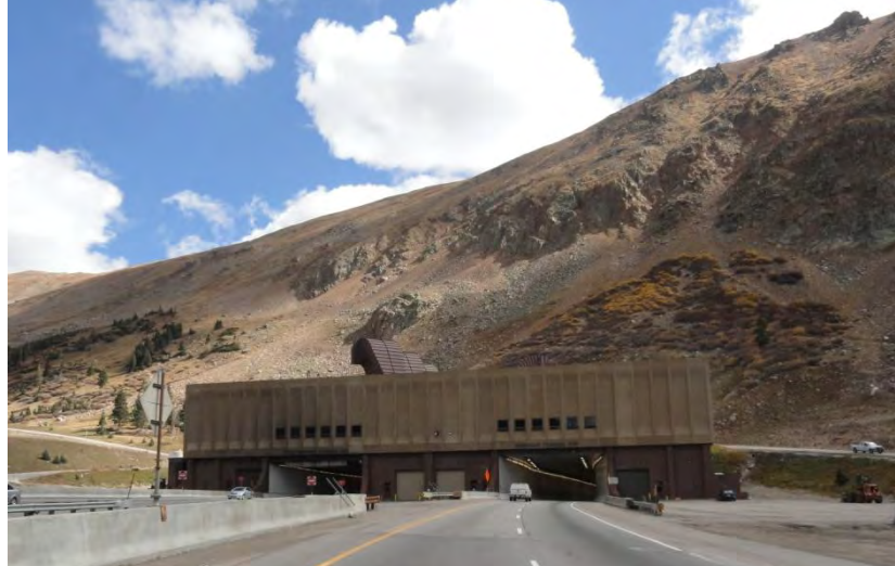
Figure 6. Eisenhower Memorial Tunnel, Colorado.
