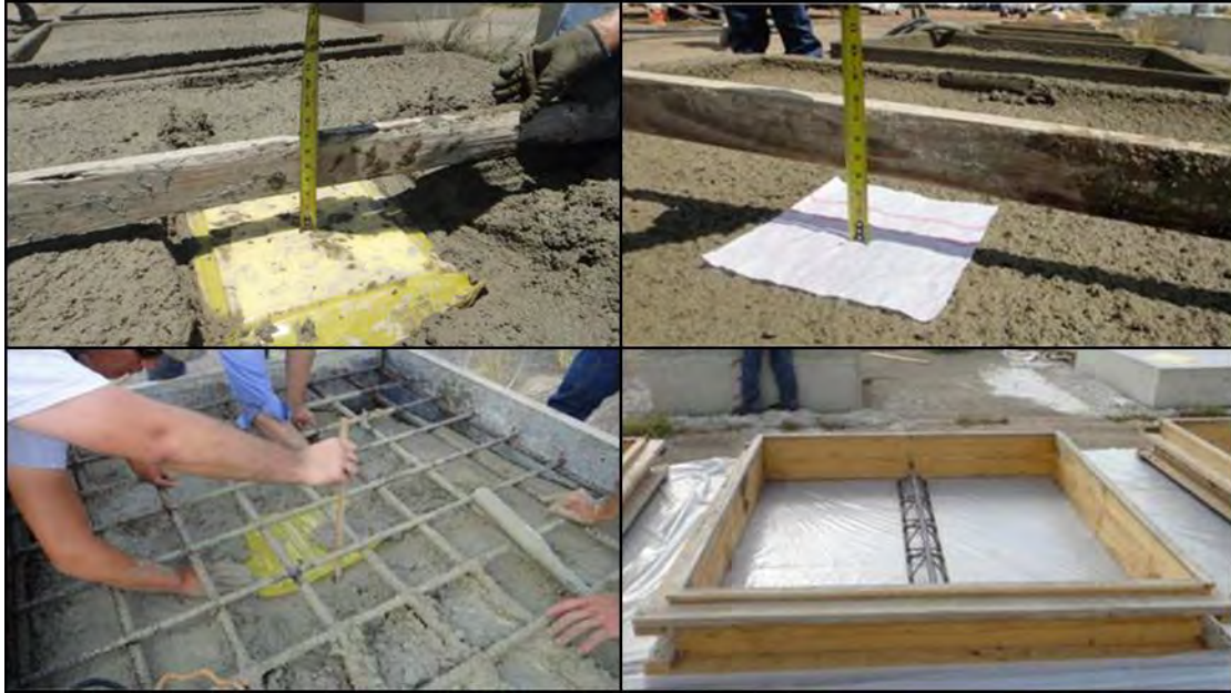
Figure 1. Construction of slabs with simulated defects.
