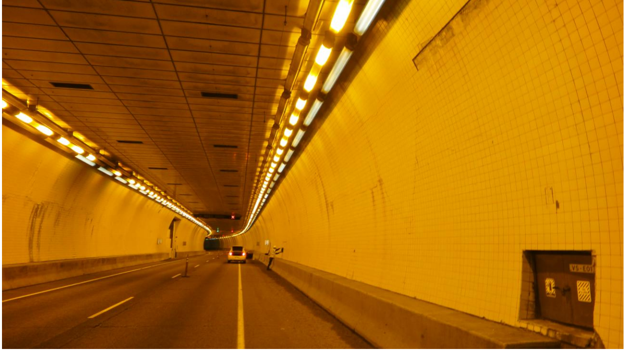
Figure L-29. Visual image of the Hanging Lake Tunnel roadway section.
