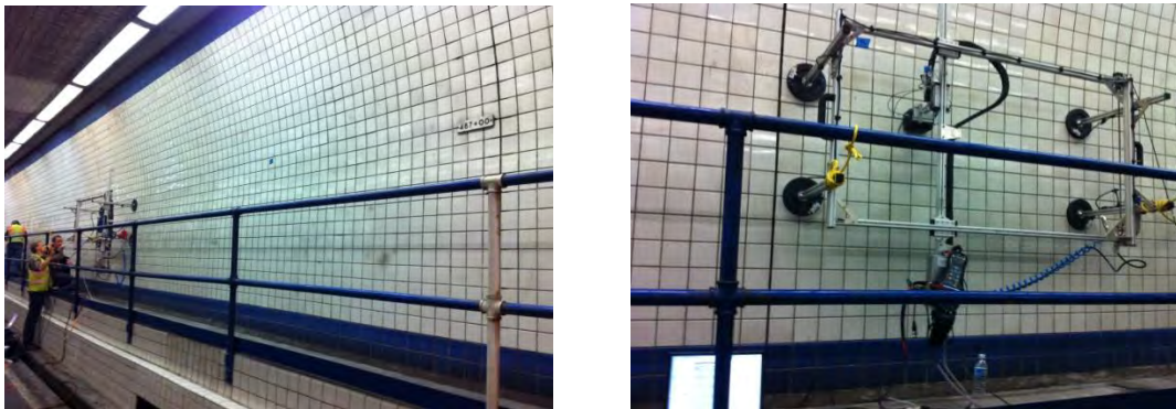
Figure Q-88. CPB4 near Sta. 486+28.
