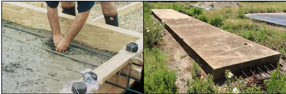
Figure 2. Clay lump slab construction.
