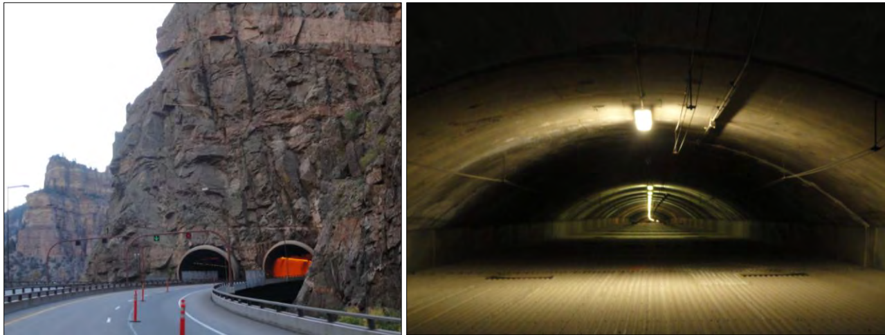
Figure M-17. Hanging Lake Tunnel: exterior (left) and interior plenum view (right).
