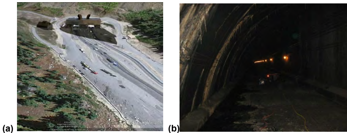
Figure Q-2. Entrance to the Eisenhower tunnel (a) and the interior of the supply air duct, where measurements took place (b).
