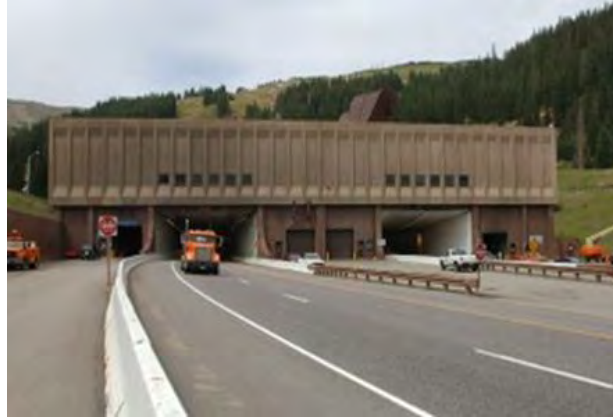
Figure P-2. Outside view of Eisenhower Tunnel.
