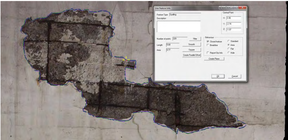
Figure X-8. Information on spalling by the ventilation shaft: coordinates of center point and area.
