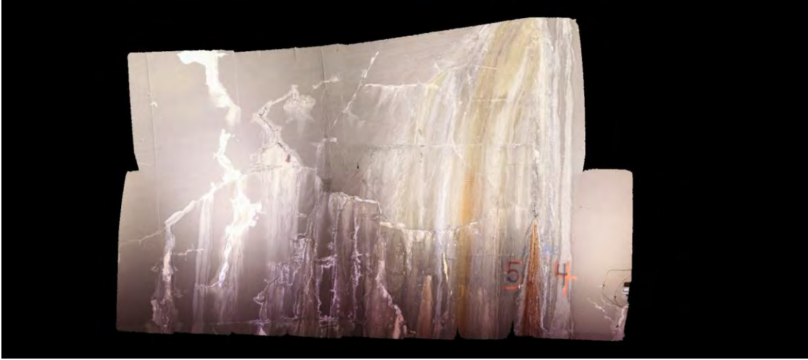
Figure X-19. Eisenhower-Johnson Tunnel: clean air supply duct south-west ventilation building: view of the south lining wall from within the duct.
