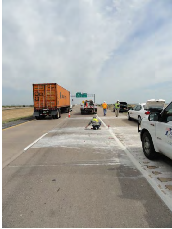
Figure M-21. I-20 in Ft. Worth, Texas.
