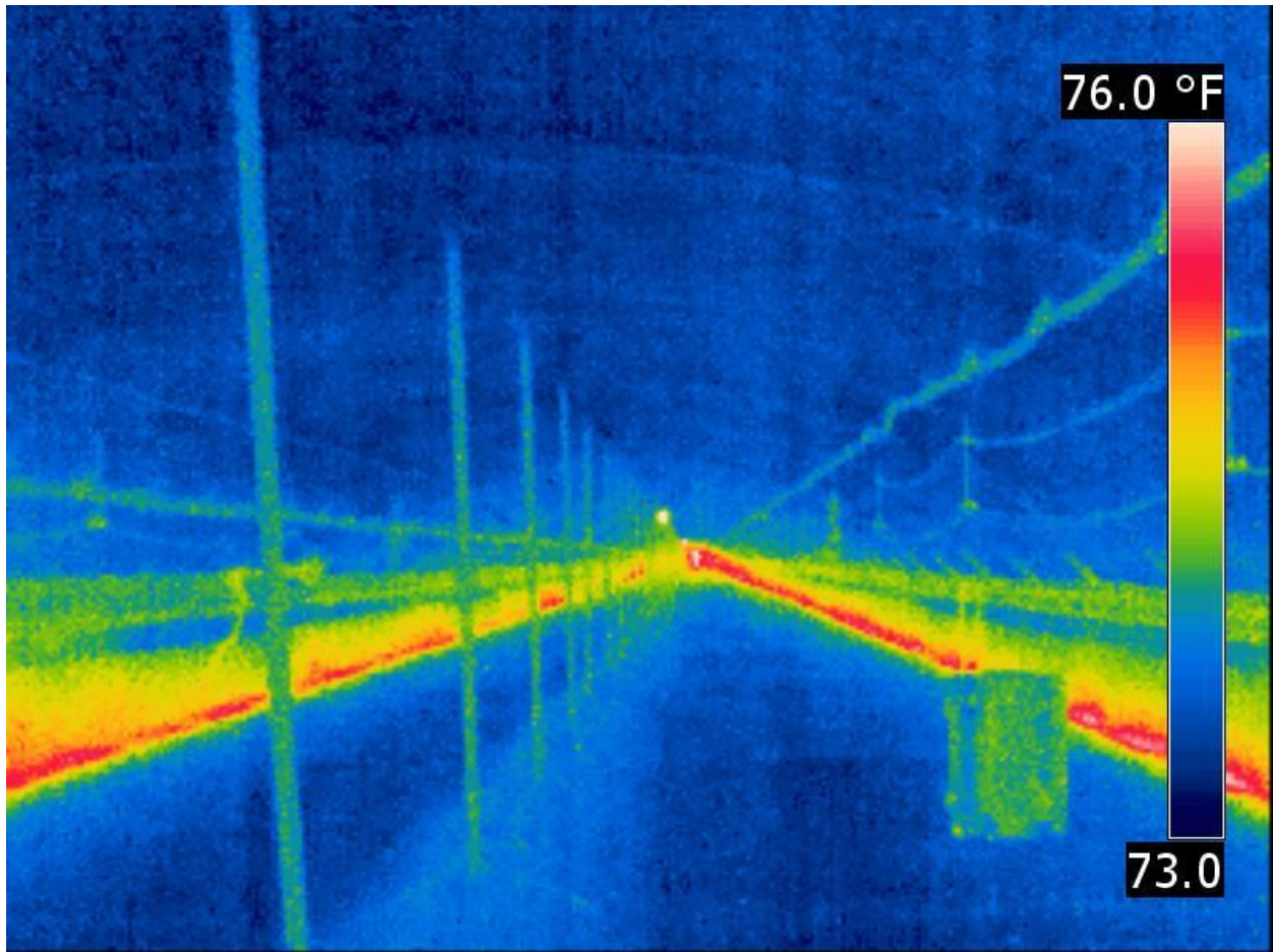
Figure L-5. FLIR T-300 infrared image of the top of the Chesapeake Bay Tunnel. The areas in red are air vents.
