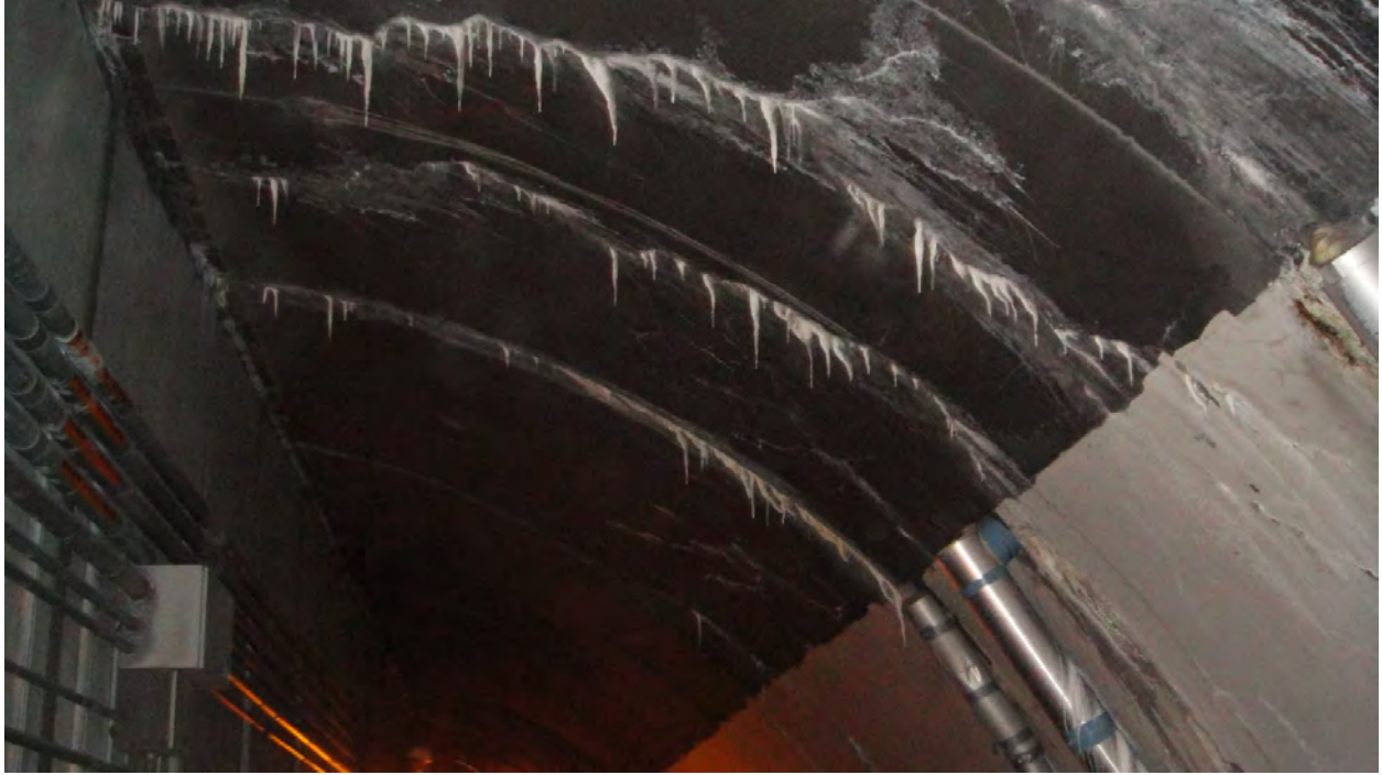
Figure L-17. Visual image of the top of the Eisenhower Memorial Tunnel.
