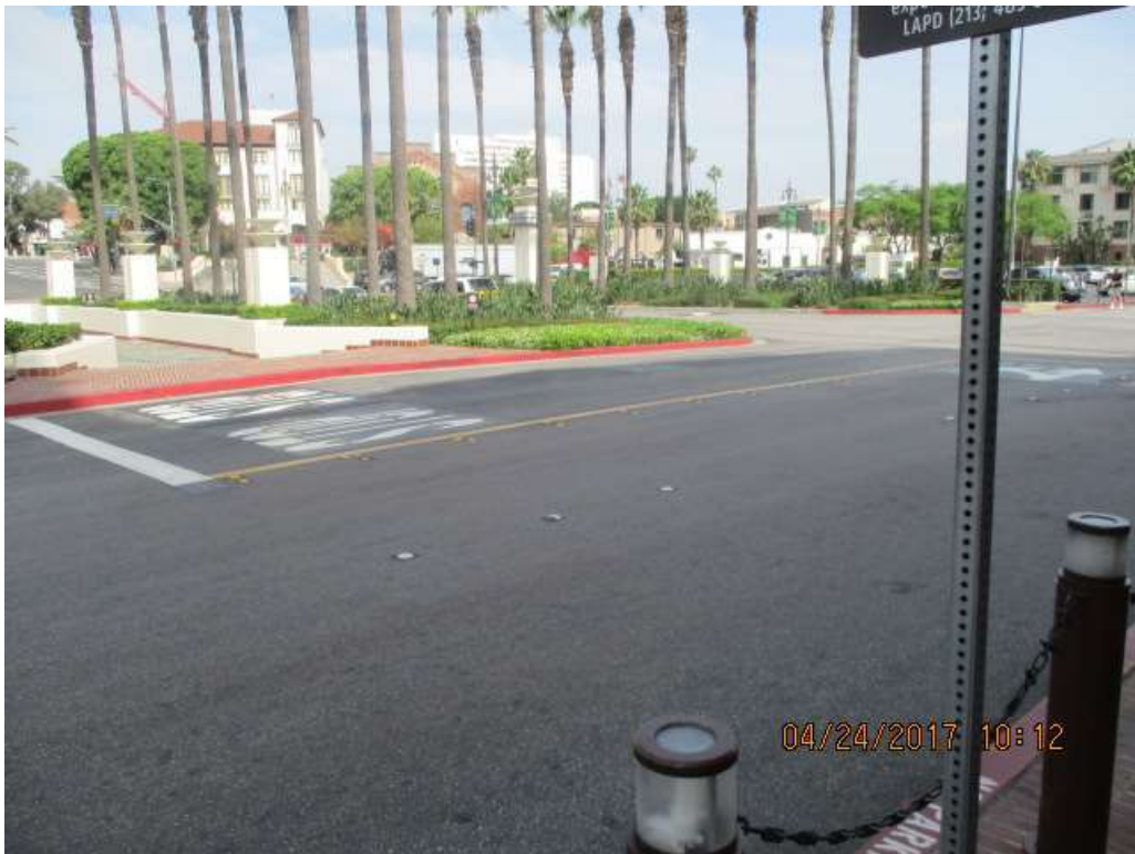
Photograph 8 - View facing northwest at the LAUS entrance and forecourt area of the Project.
