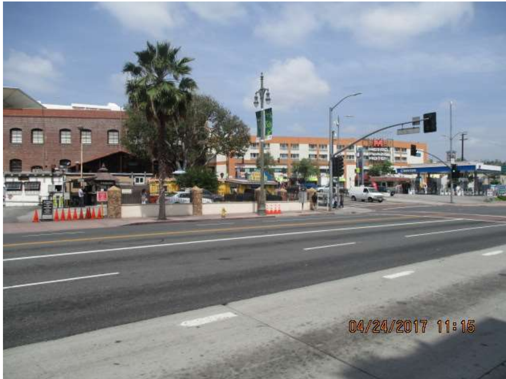
Photograph 13 - View of intersection of Alameda Street / Cesar Chavez, and the properties located at the northwest (Chevron gasoline station, right)) and southwest (former gasoline station, left) corners.
