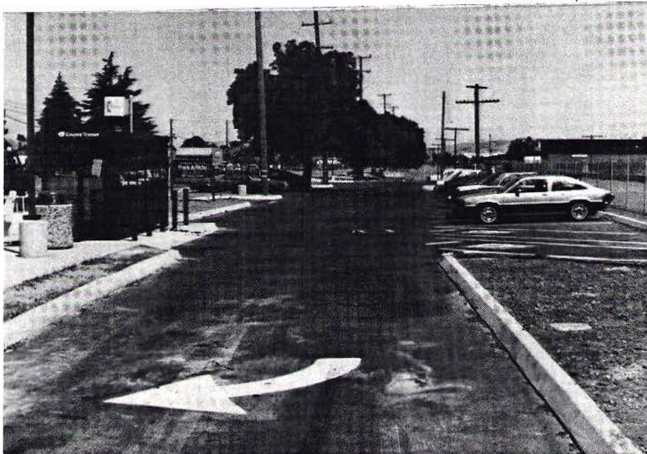
Fig. 2 - Park-and-Ride Lot Built by Santa Clara County Transit District for Express Bus Lines to San Jose
