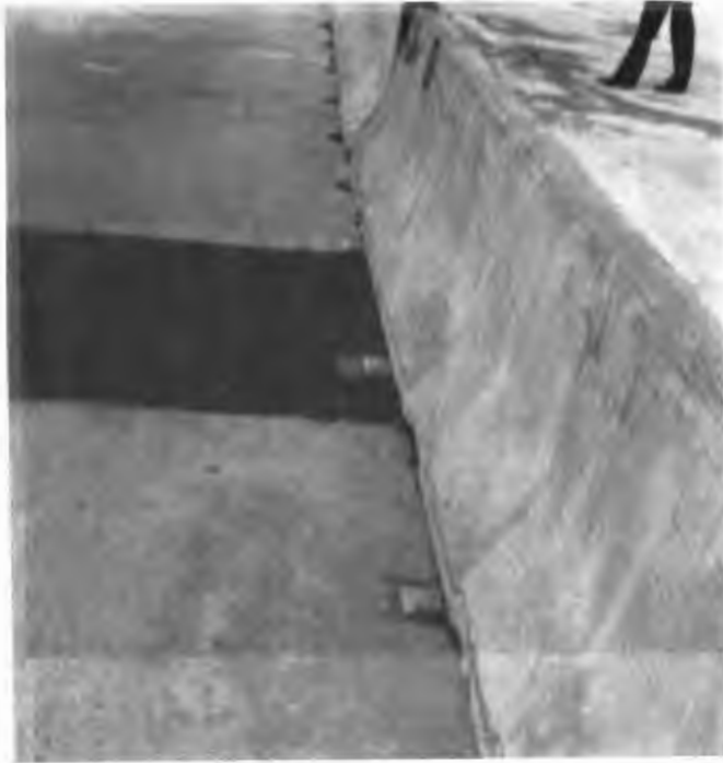
Pavement marker on pavement close to barrier
