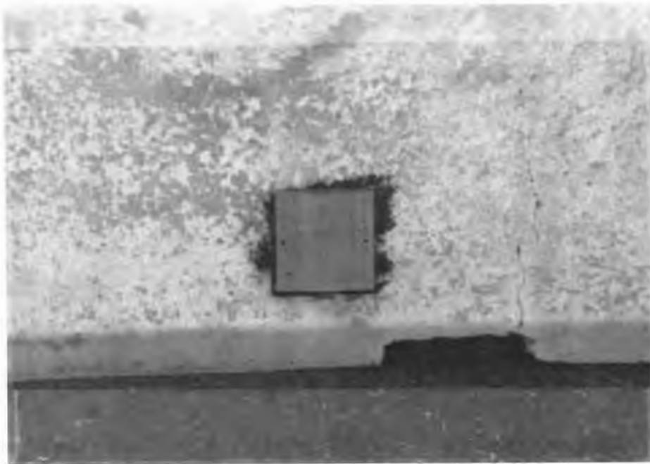
Pavement marker on face of barrier
