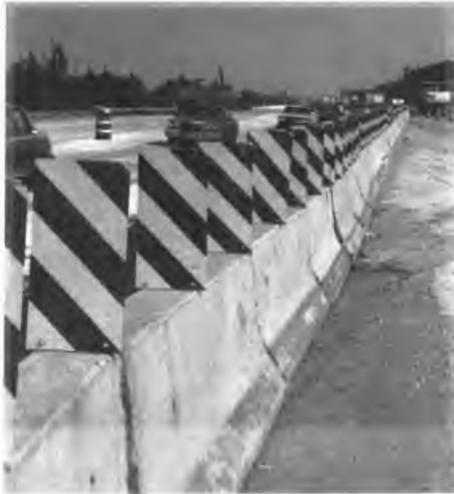
Figure 6. Delineating with vertical panels
