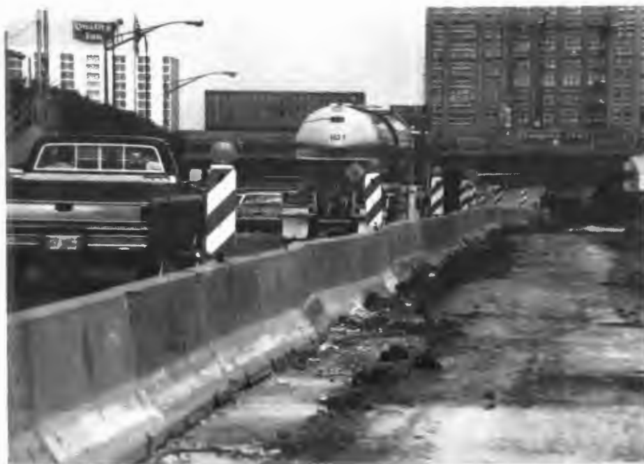
Figure 13. Combined use of warning lights and vertical panels
