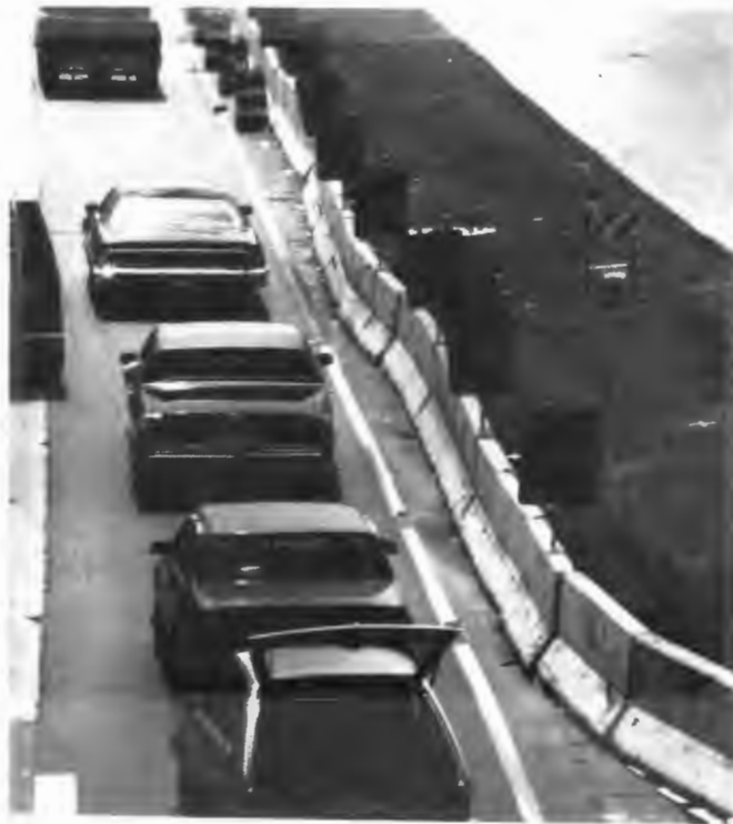
Figure 7. Delineating with chevron arrows (Application not recommended by the MUTCD)
