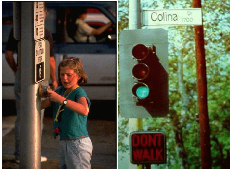
Figure 11. On some high-volume or multi-lane roads, traffic and pedestrian signals are needed to better accommodate pedestrian crossings.
