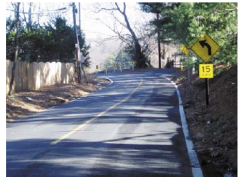
Photo 6 - Obscure or otherwise difficult to see signs. Also, signs may be incorrectly placed, limiting their intended effectiveness.
