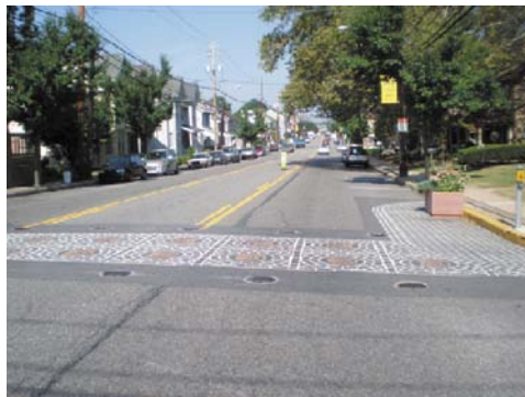
Photo 7 - New crosswalk markings that allow communities flexibility in materials and design are approved for use by PennDOT.
