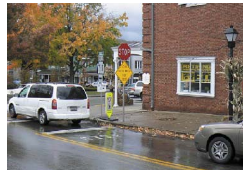
Photo 3 - Improperly used crossing signs. The stand-alone pedestrian sign should be on the centerline in advance of the crosswalk.
