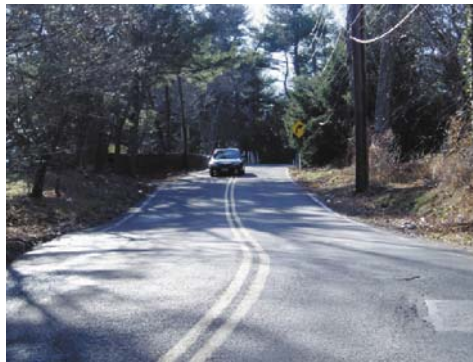
Photo 4 - Winding roads, particularly when narrow, are difficult for drivers to negotiate while remaining within their lane.
