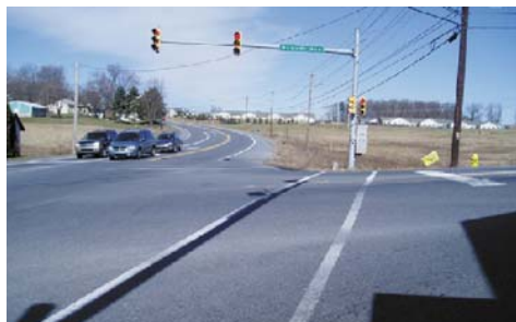
Photo 2 - A long crosswalk that seems to go nowhere. Crossing times for the elderly, for children, and for special needs persons will be long. Also, the parallel lines crosswalk marking is common, but may not be as visible as other crosswalk markings.
