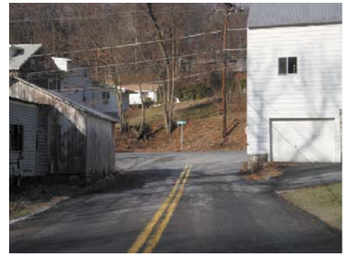
Photo 5 - Narrow or non-existent clear zones
