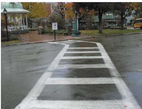
Photo 1 - Unusual crosswalk that may cause difficulty for drivers to predict pedestrian movements
