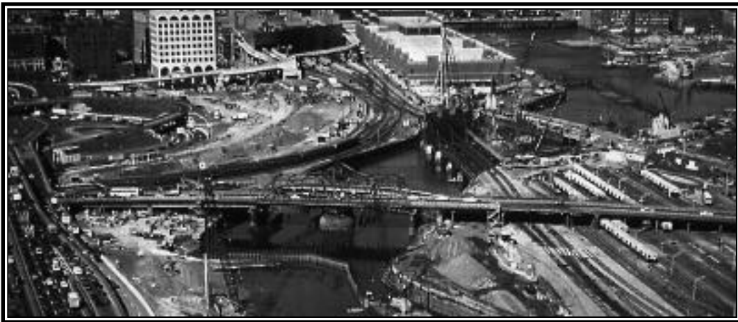
Central Artery/Third Harbor Tunnel Project, Boston, MA.
