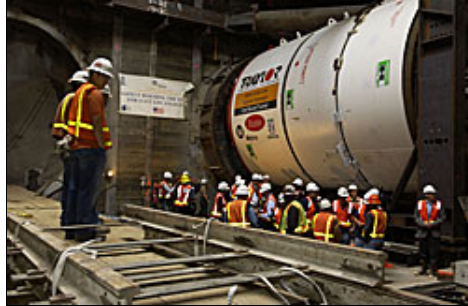
Fully assembled underground, each tunnel boring machine will weigh more than 2 million pounds and stretch 344 feet. They will carve 21-foot diameter tunnels and install pre-cast concrete tunnel liners.
