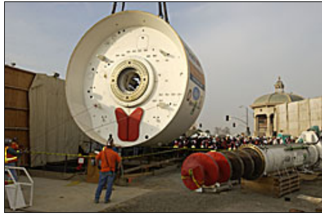
Machine is lowered into shaft at First and Boyle streets. Marachi Plaza is in the background.
