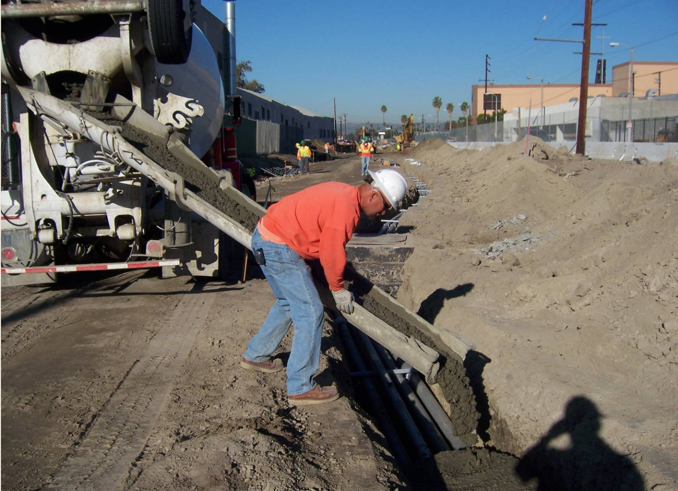
Installation of 6-Way Ductbank in Segment B
