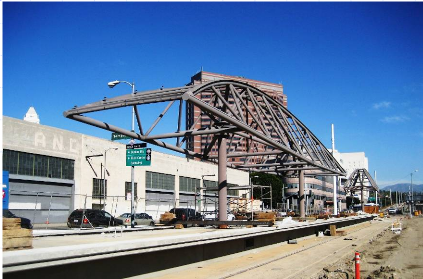
Little Tokyo/Arts District Station - Northeast corner of 1st/Alameda.
