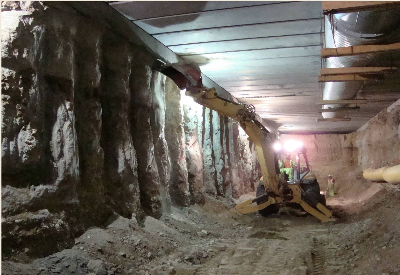
Continued Excavation of Trench Structure
