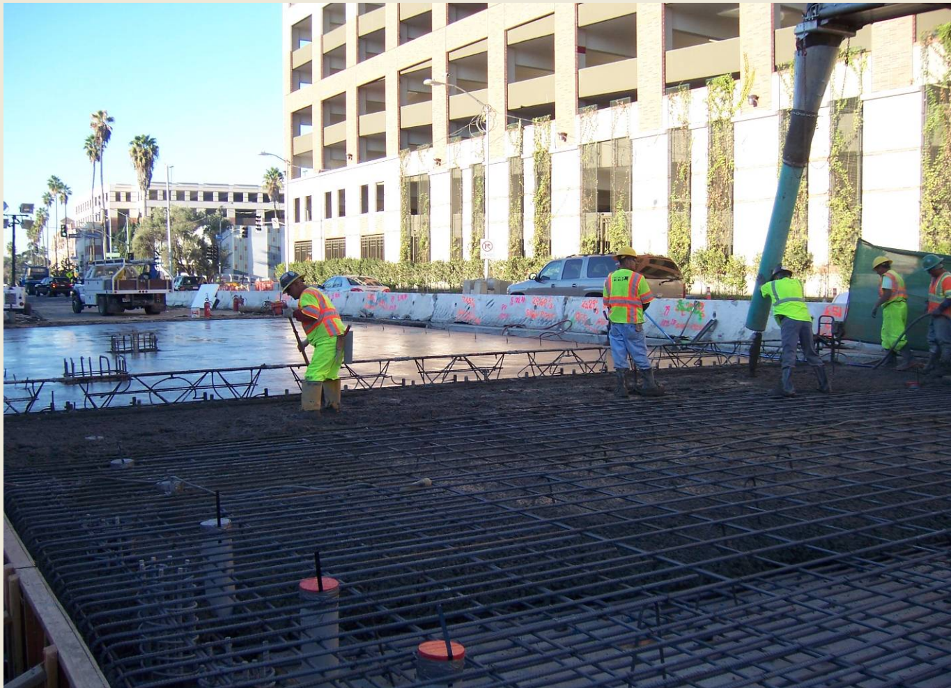
Trench Structure Roof Slab Concrete Placement
