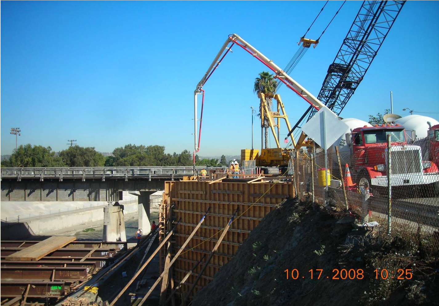
National Blvd Bridge Abutment 1 Concrete Placement
