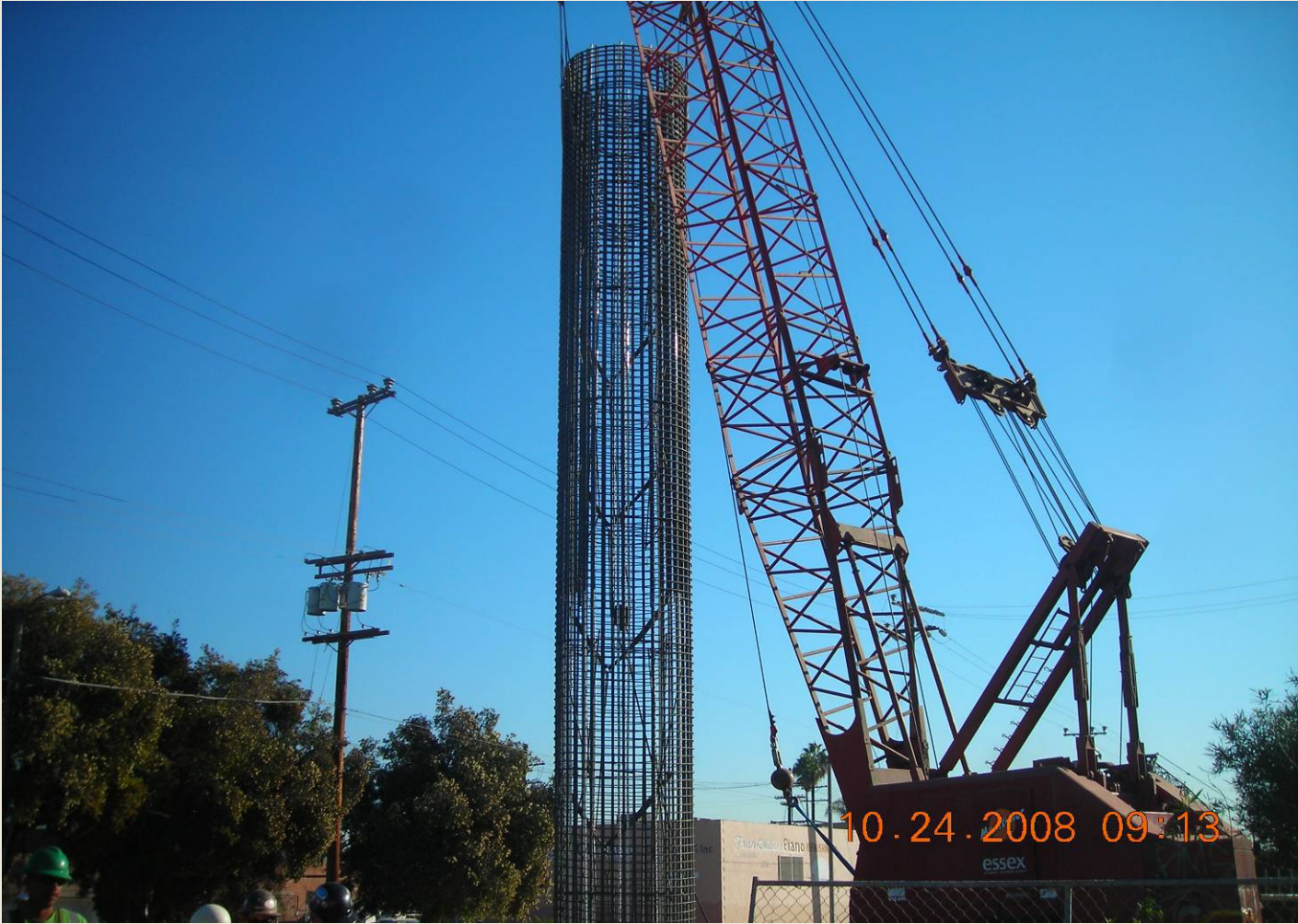
La Brea Aerial Structure CIDH Pile Installation
