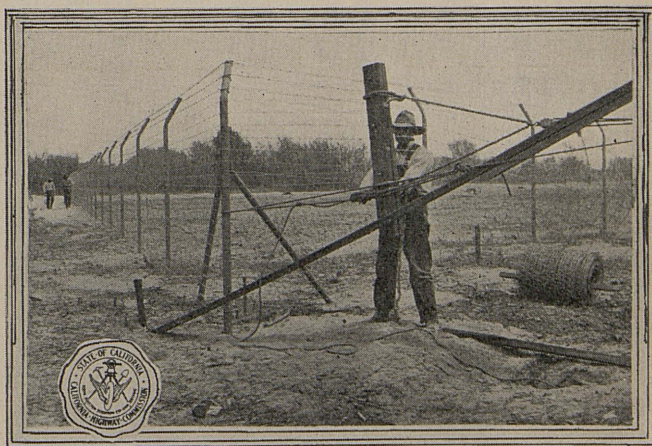
DISCARDED PIPE NOW FENCE POSTS—Division VII uses discarded pipe for fence posts when enclosing maintenance yards. The pipe is secured from the Lankershim shop. The view above shows the fence being erected at the new Santa Clara River station. This type of post has proved satisfactory.
