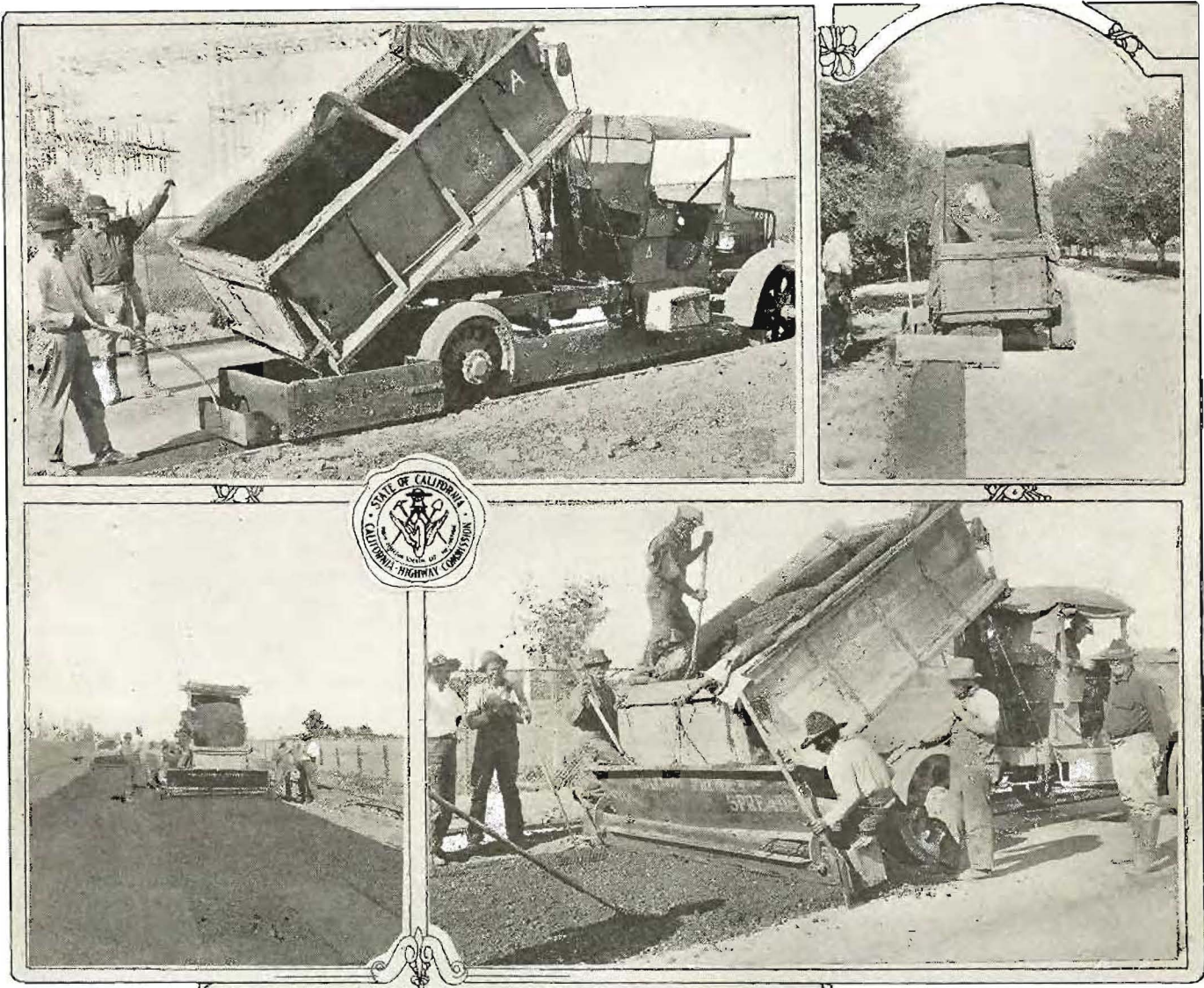
VACAVILLE WIDENING CONTRACT --Views on the Force and Curriegan asphalt contract, Solano County, where a new plan for widening the fifteen-foot concrete pavement with asphalt concrete is being tried out. Upper left, method used to spread asphalt concrete mix in shoulder trench for widening the pavement to twenty feet. Upper right, spreading the two-foot gravel shoulders along completed pavement. Lower views show spreader used in placing asphalt concrete mix over old concrete pavement and new shoulders. Use of labor-saving devices has been a feature of this job. (Div. X.)
