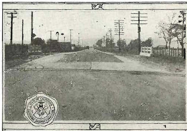
Widening the highway with flush concrete shoulders—a view taken immediately west of Fairfield, Solano County, Division X. The bridge at this point also was widened and a new railing erected. A gasoline tax job.
