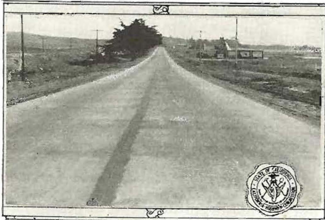
New cement concrete pavement on the Jahn and Bressi contract, in San Diego County, showing center expansion joint. A gasoline tax job.
