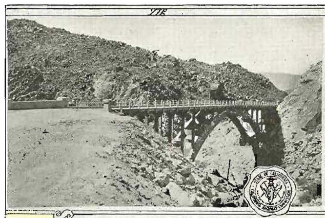
Myers Creek bridge at the foot of the Mountain Springs Grade, Imperial County, on the state highway between San Diego and El Centro.
