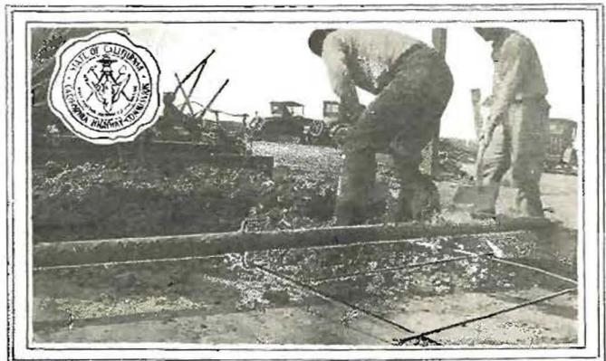
ANOTHER DIVISION VII INVENTION IN USE—Device perfected by resident engineers to hold cement concrete pavement reinforcement in position during placing of mix.
