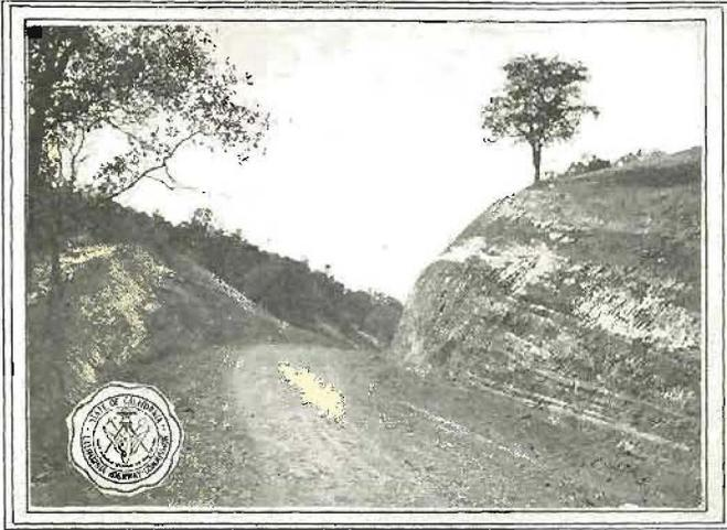
BROKEN SLOPES—View on convict job in Lake County. Division I, showing (on right of cut) broken slope which saved grading quantities.
