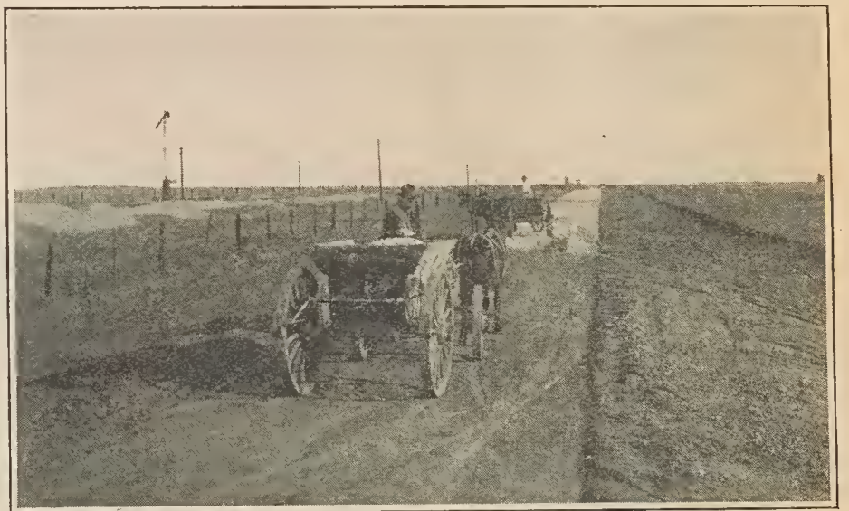
Building the State Highway Near Marysville.
