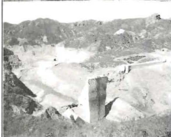
Upper left, The St. Francis reservoir before the collapse of the dam. Lower left, Scene at the dam site following the failure of the structure. Note the portion of the dam left standing and the white markings on the stream bed which denote the height that the water reached as it rushed down the stream. Upper right, Scene at brow of west wing showing cross-sections of formation upon which dam was built.
