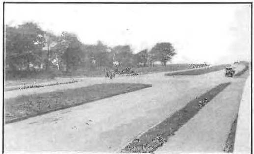
Section of finished roadway on the Glasgow end. Sidewalks are of tar macadam. After the Telford base is thoroughly locked and filled, the road is surfaced with three inches of tar and macadam.
