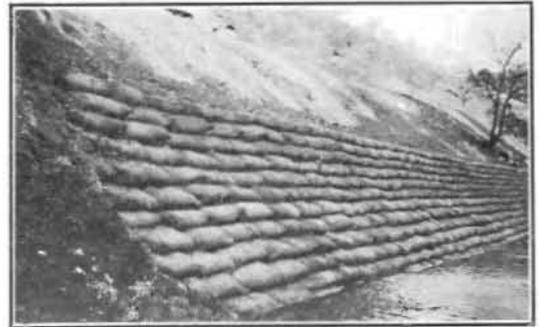
Sacked concrete riprap protecting embankment of newly constructed 24-foot graded roadbed in Lake County, a portion of the Ukiah-Tahoe state highway.
