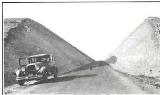
This second picture is that of the large cut lying just to the west of the large fill above mentioned and from which material was obtained to construct the fill. The cut has a maximum depth of 66 feet and approximately 80,000 cubic yards were removed, all of which was used to construct the fill. This large cut and fill are portions of a line change about three miles in length, which shortened the distance between Bakersfield and Kern Canyon by one-half mile.
