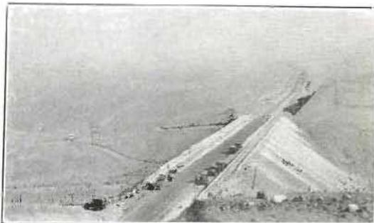
The above view is that of a large fill on Kern River road about 10 miles east of Bakersfield which has recently been completed. The fill has a maximum height of 77 feet and was constructed mostly by sluicing. This section is on the Santa Maria to Freeman highway via Bakersfield and Walker's Pass.
